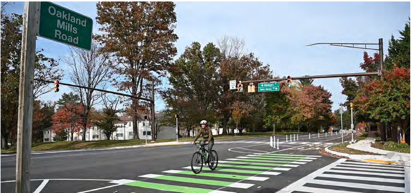
The County finished a Complete Streets project on Oakland Mills Road between Old Montgomery Road and Dobbin Road. The reconfiguration of the roadway improved safety for drivers, pedestrians and cyclists.
