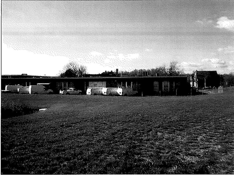
Rear elevation looking west
