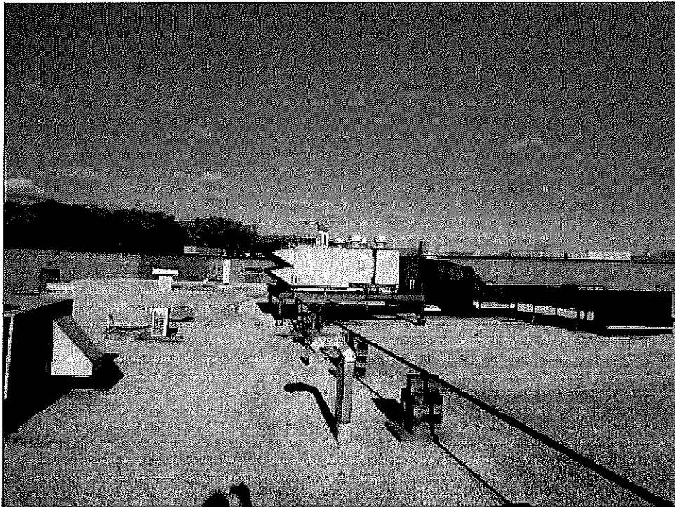
Subject roof showing HVAC equipment looking north towards Atholton High School
