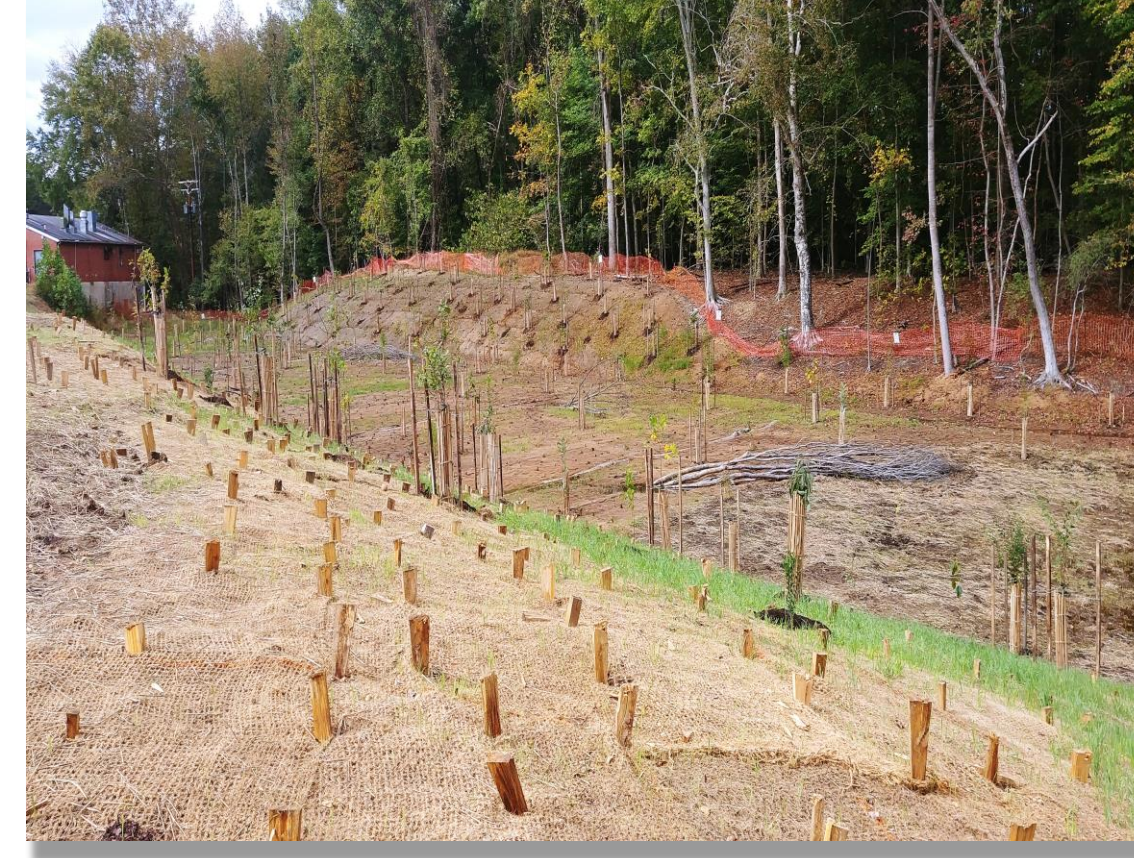
IMMEDIATELY AFTER CONSTRUCTION
