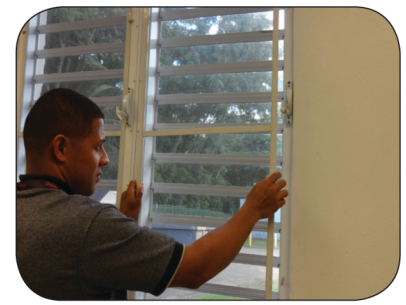
Install or repair window & door screens.
