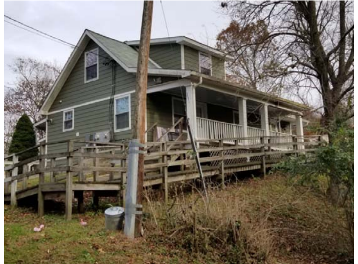
Figure 9 - West side of the house (original front of the house)
