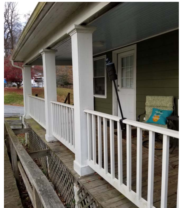
Figure 10 - Existing front porch and columns
