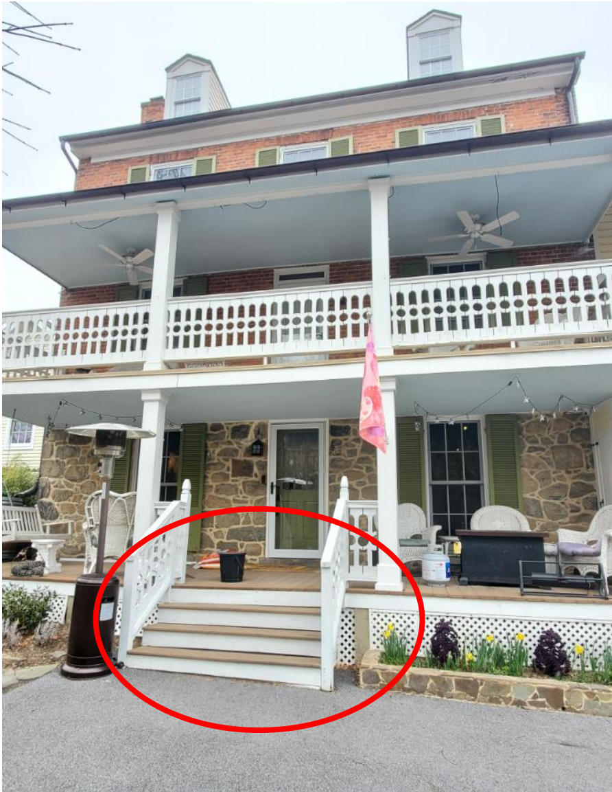
Figure 30: Steps light to be installed on main house porch stair riser every other step.
