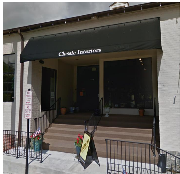
Figure 19 - View of recessed area
