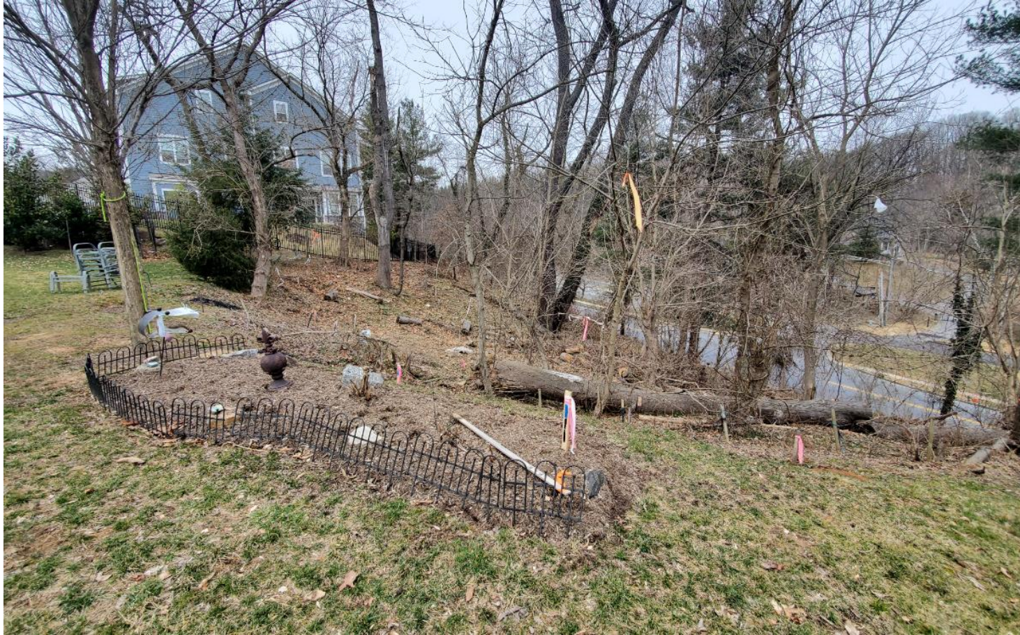
Figure 37: Location of proposed Northeast retaining wall. Ellicott Mills and Burgess Mill are visible in the distance.
