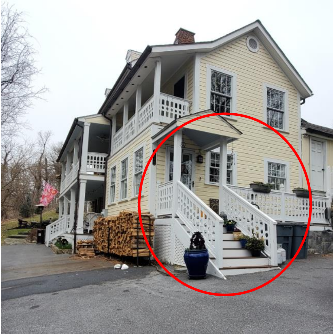
Figure 28: Steps light to be installed on kitchen porch stair riser every other step.
