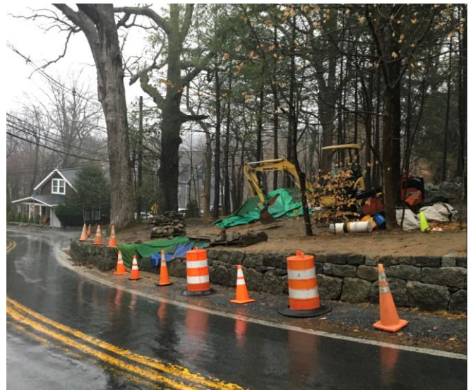
Figure 7 - Realigned wall. Note the increased width of the shoulder.
