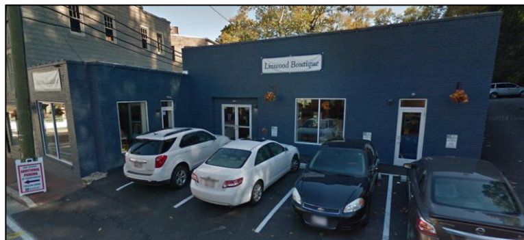
Figure 10: 3709 Old Columbia Pike, front of building.
