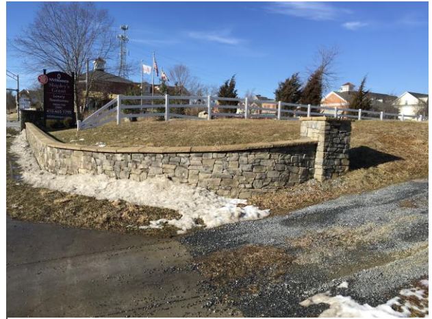
Figure 6: Existing stone wall at west exit.
