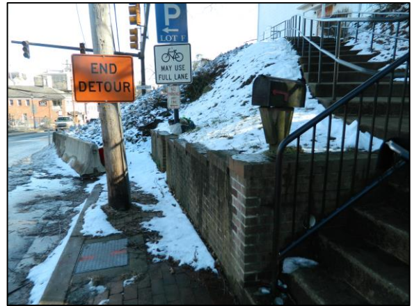
Figure 13: St. Luke AME Church existing brick wall on northwest side of property.
