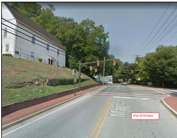
Figure 11: St. Luke AME Church slope prior to the 2016 flood.
