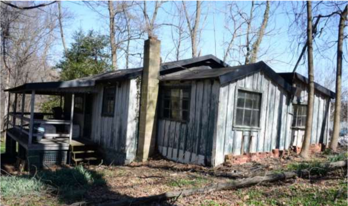
Figure 16 - View of building
