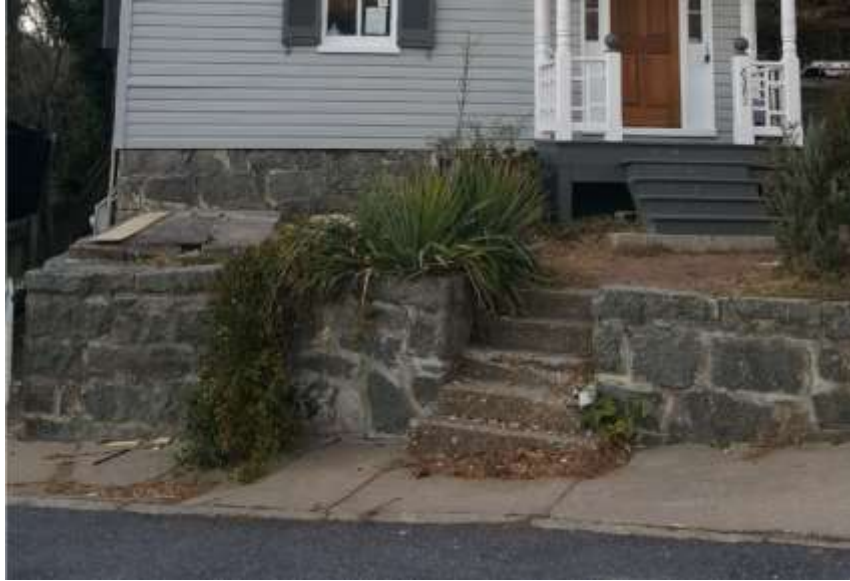
Figure 40 - Front steps and retaining wall
