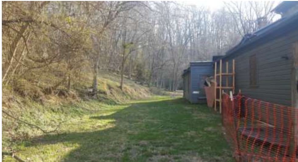
Figure 8- View behind house
