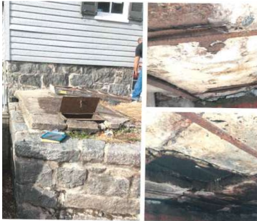
Figure 41 - Concrete slab
