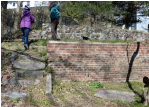
Figure 45 - Rear retaining walls
