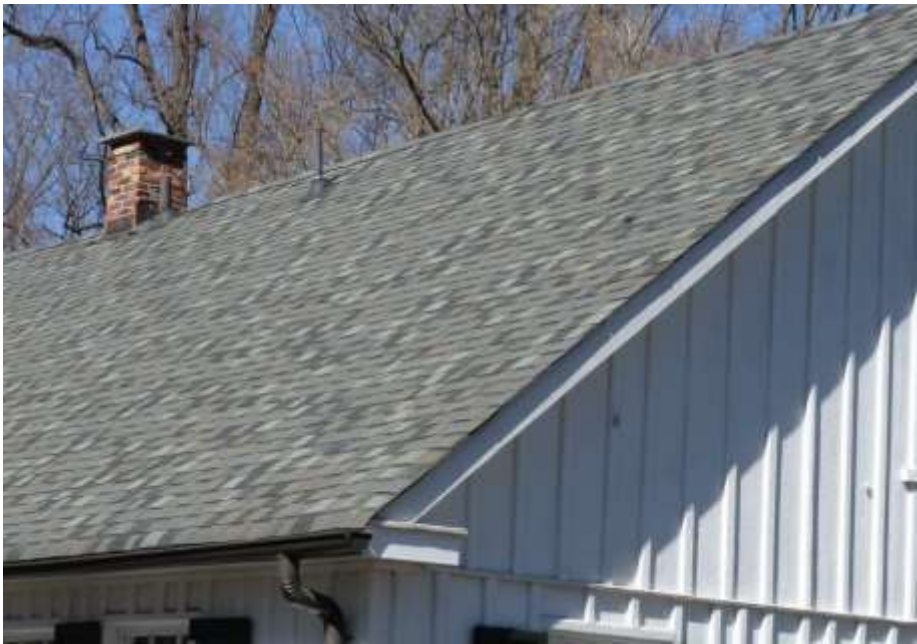
Figure 17 - Roof on main house
