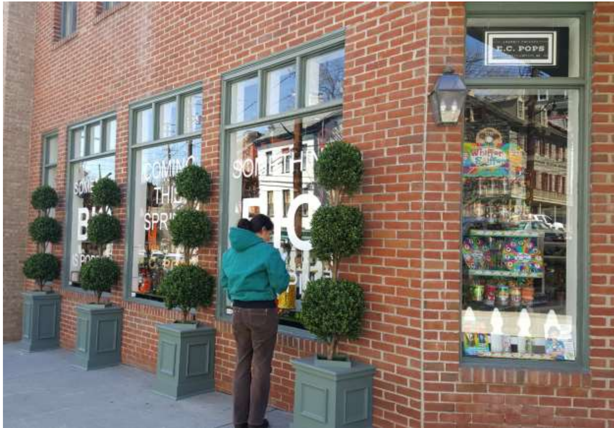
Figure 11 - Front of building
