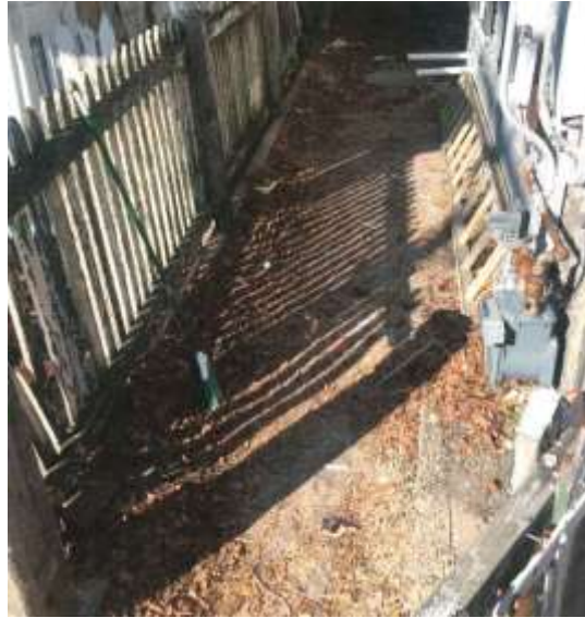
Figure 42 - Brick side walkway
