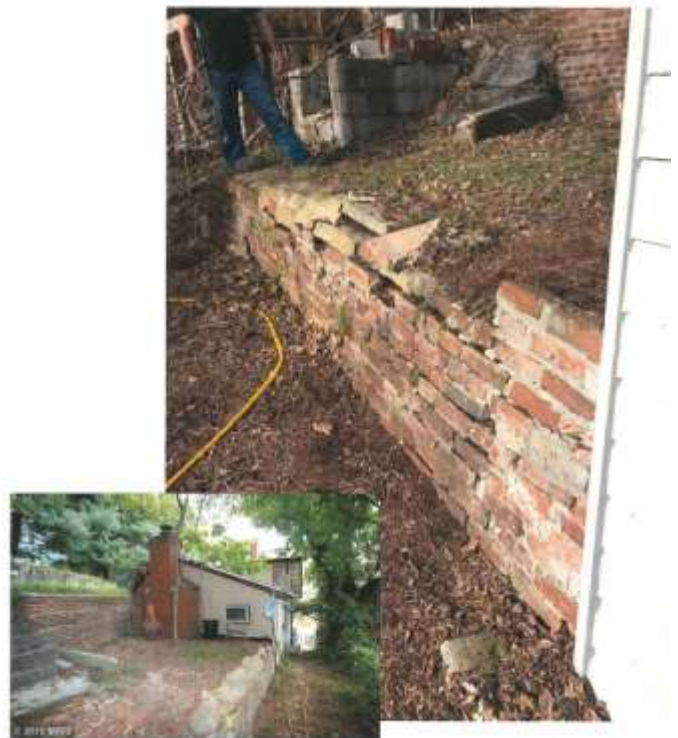
Figure 46 - Rear retaining walls
