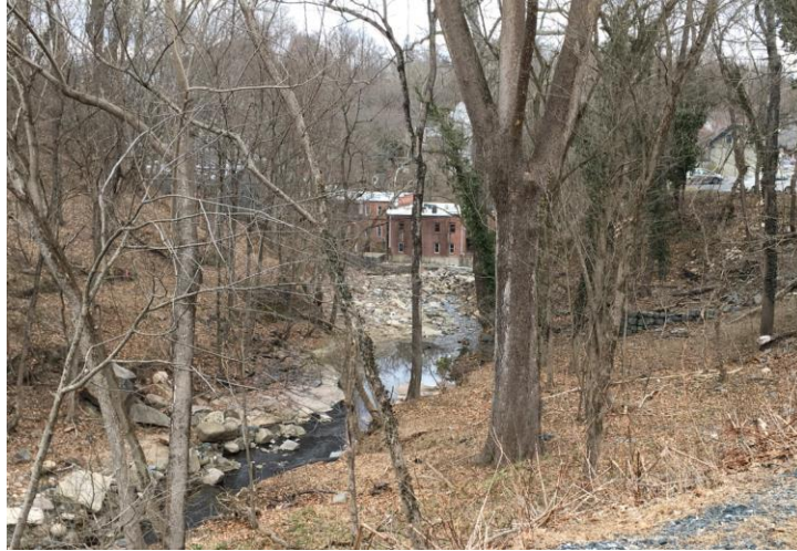
Figure 3 - View looking down New Cut stream at the rear of buildings along Main Street
