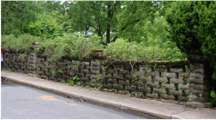
Figure 9 – Previously existing wall
