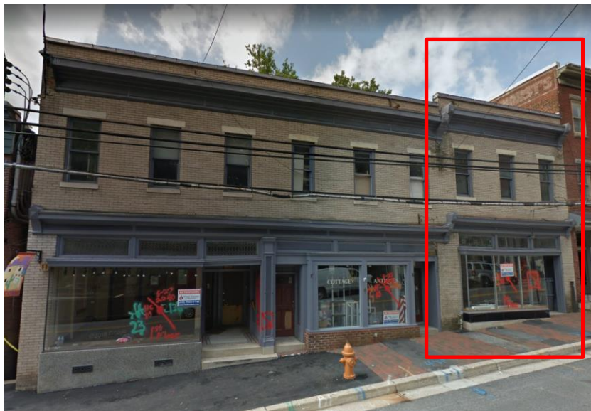
Figure 13 - Buildings located at 8173, 8181 and 8185 Main Street (in red box)
