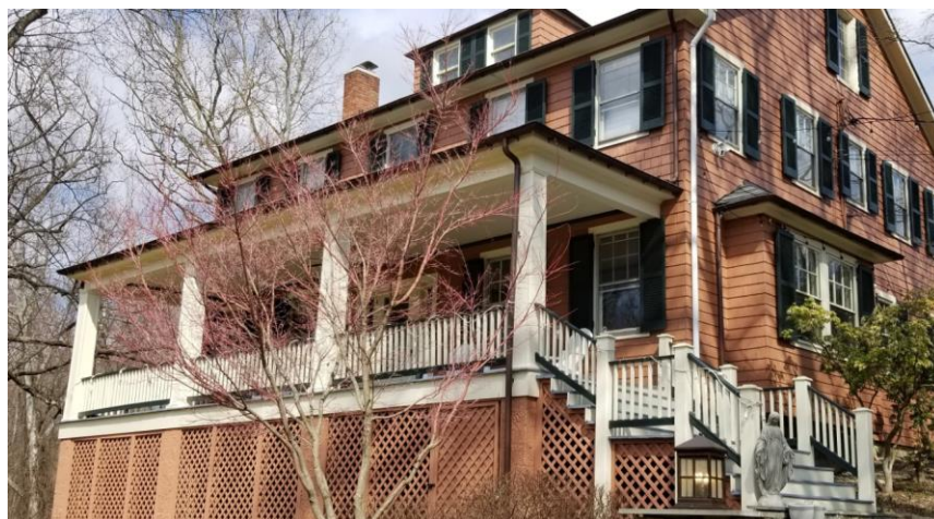
Figure 11 - View of gutters and downspouts
