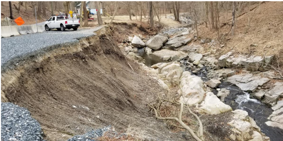
Figure 4 - Looking up New Cut Road
