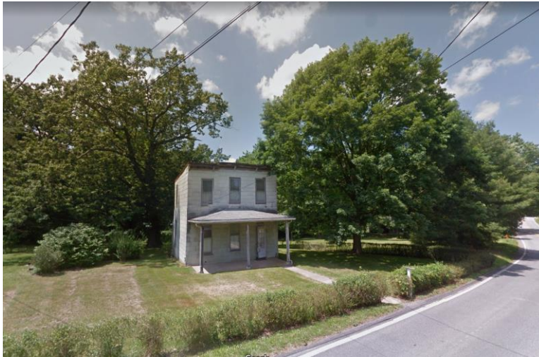
Figure 12 - Historic house to be demolished
