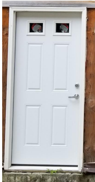
Figure 24 - Existing door at 8181 Main Street
