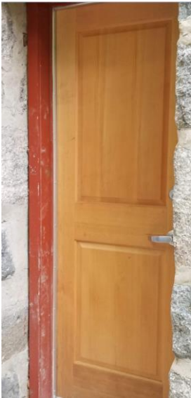
Figure 23 - Existing door at 8185 Main Street
