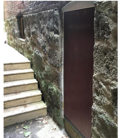
Figure 26– Existing door covering and window on side alley at 8173 Main Street
