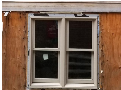
Figure 28 - Existing vinyl windows at 8181 Main Street
