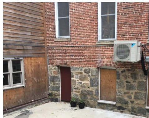
Figure 32 - View of stone foundation at 8173 Main Street
