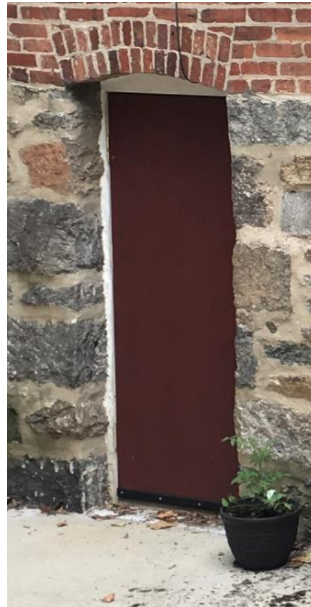
Figure 25 - Existing door covering at 8173 Main Street
