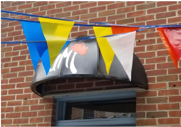
Figure 12 - Awning over door
