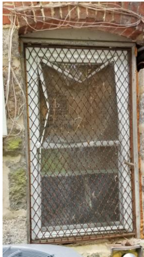
Figure 29 - View of window at 8185 Main Street
