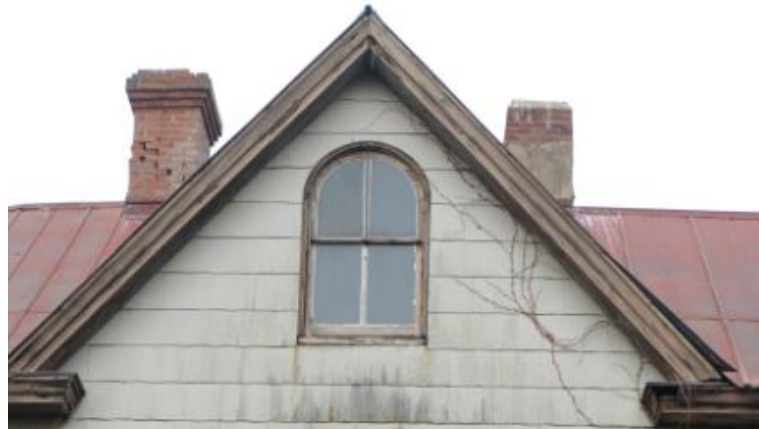
Figure 18 - View of chimneys
