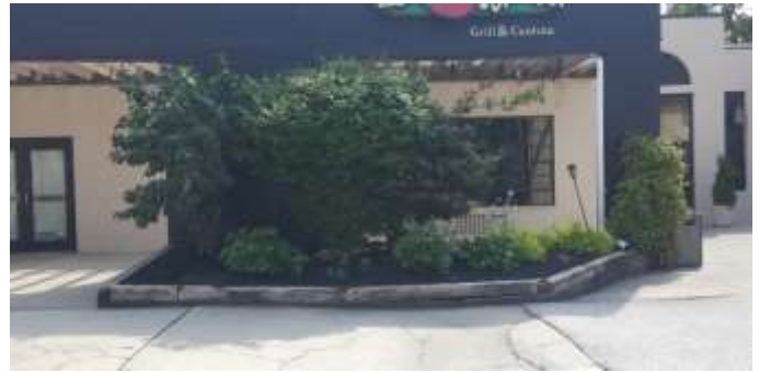
Figure 8 – Wood retaining wall to be removed
