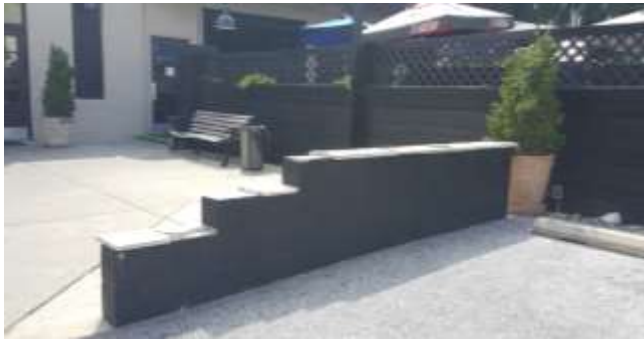
Figure 7 - Concrete block wall to be removed
