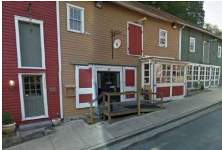
Figure 21 - Existing front ramp and stairs
