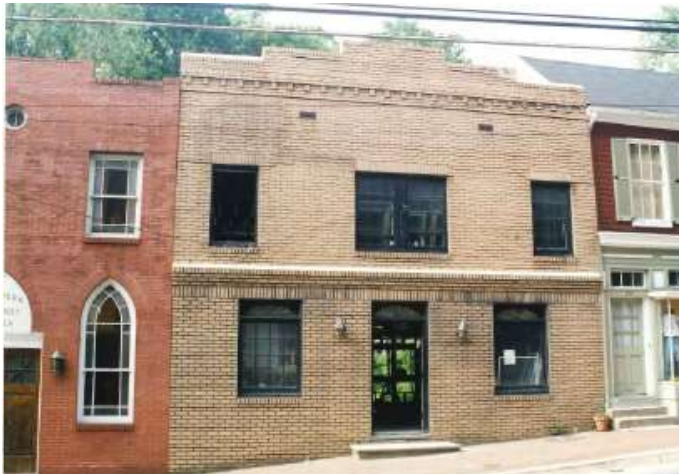
Figure 22 - Older photos of front facade
