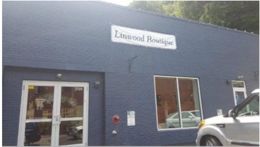
Figure 21 - Temporary banner on facade
