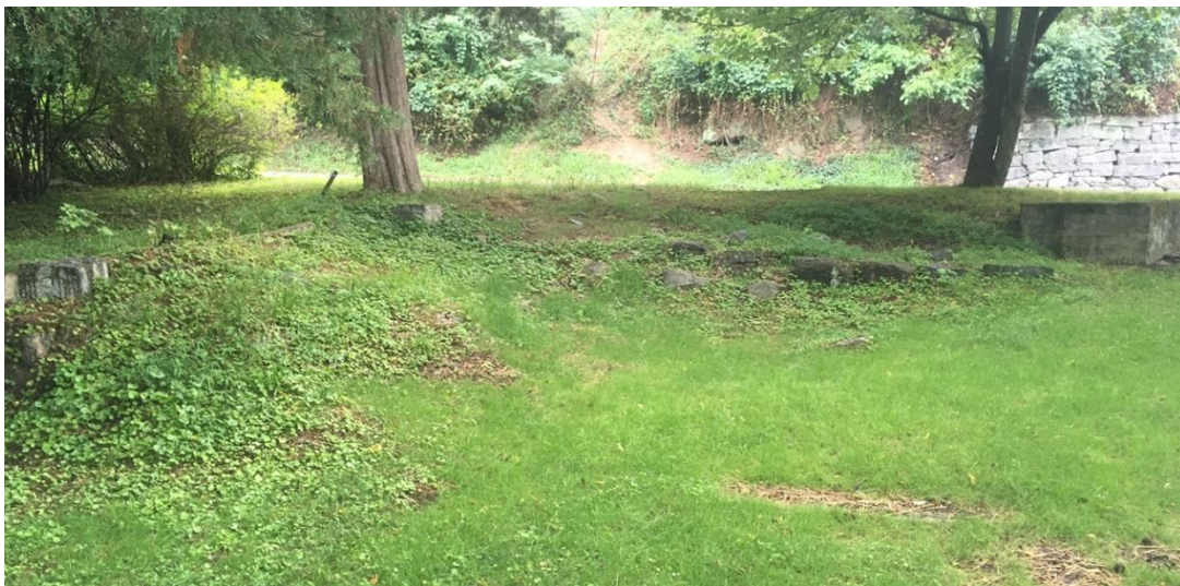
Figure 15 - Old foundation wall
