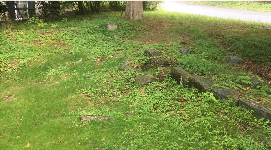
Figure 13 - Old foundation wall
