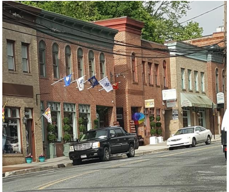
Figure 19 - Street view of building
