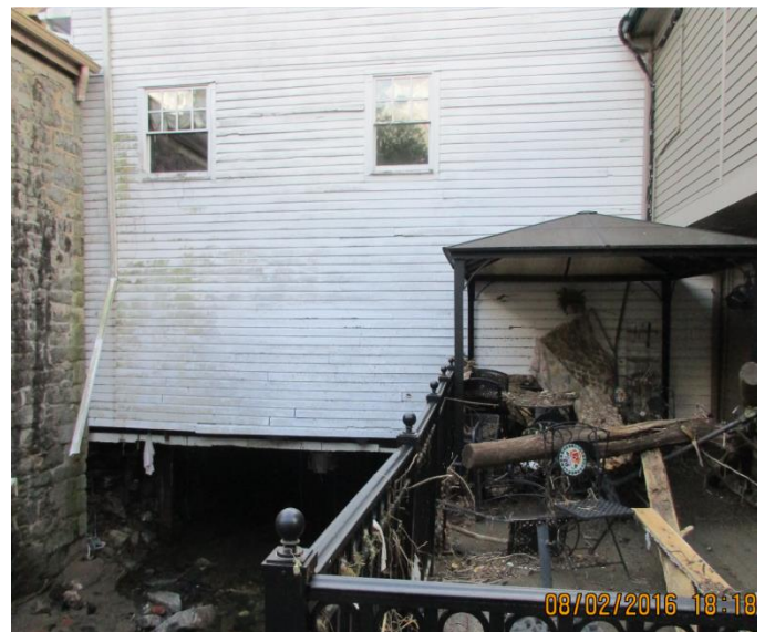
Figure 4 – East side of building in August 2016
