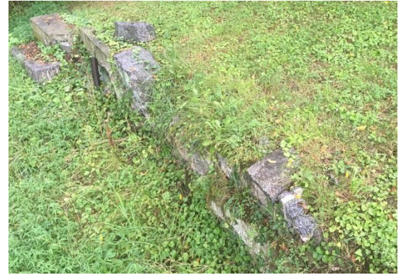
Figure 14 - Old foundation wall
