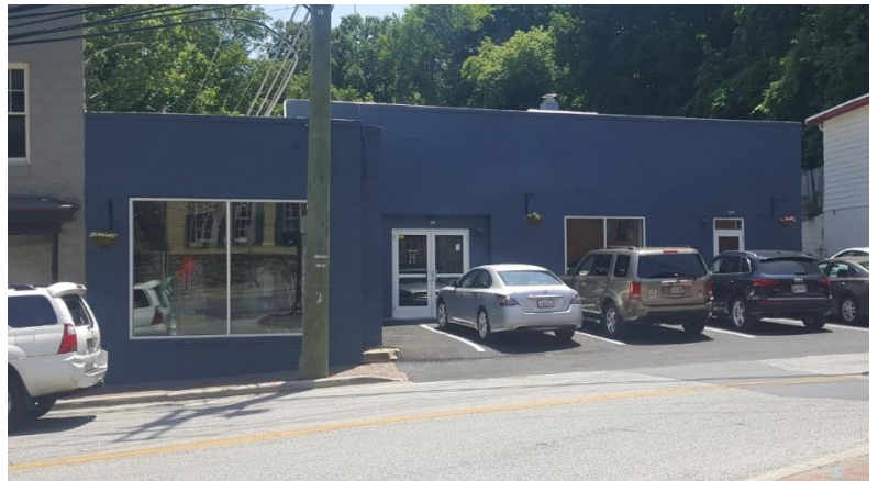
Figure 22 - Street view of building
