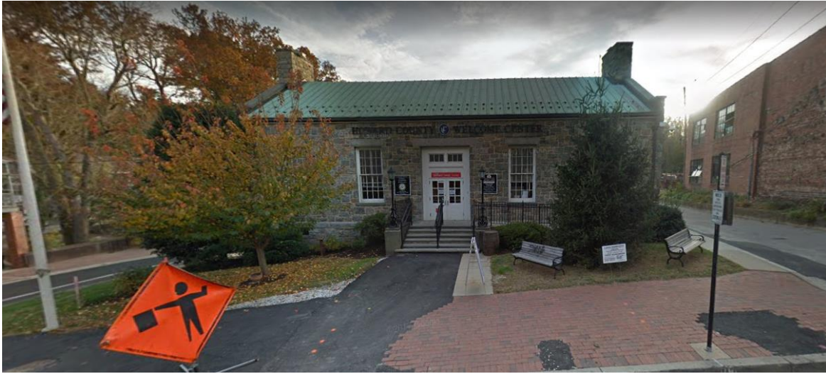
Figure 9 - Front of Visitor's Center
