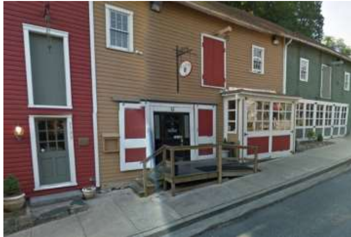
Figure 21 - Existing front ramp and stairs
