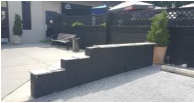
Figure 7 - Concrete block wall to be removed
