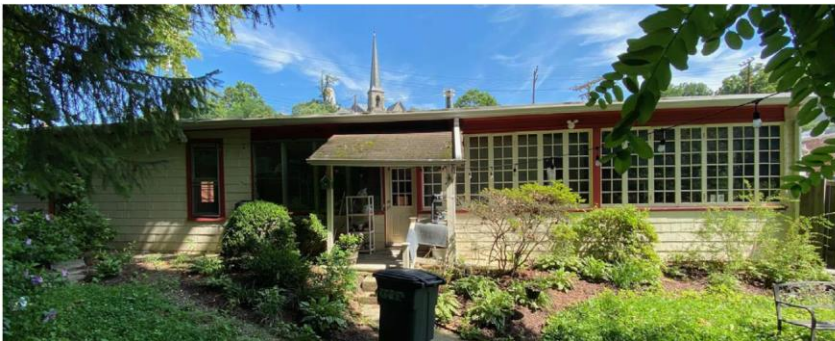
Figure 17 - Existing rear view
