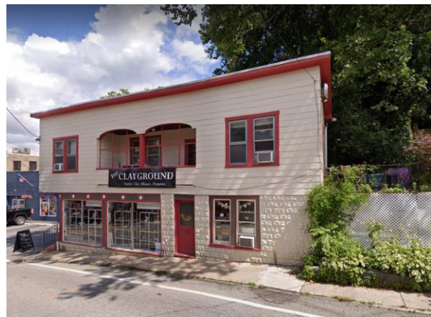
Figure 13 - Front facade along Old Columbia Pike.
