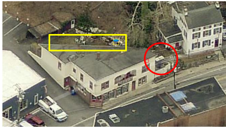
Figure 12 - Red circle indicates location of side addition. Yellow box indicates area of rear alterations.
