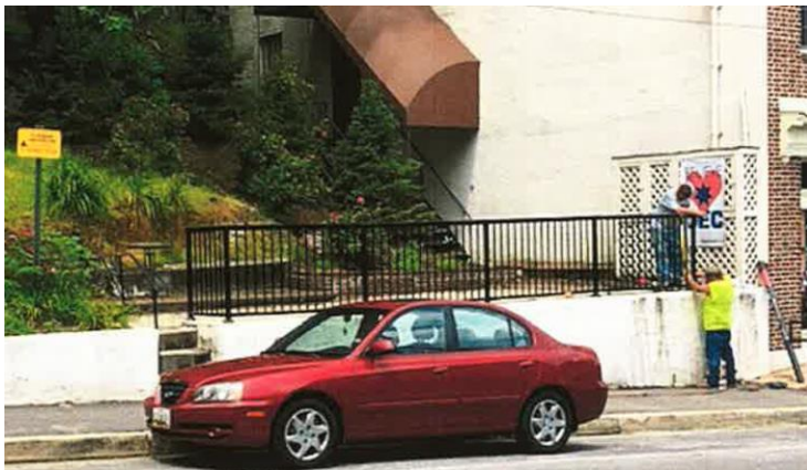
Figure 22 - Fence installed and approved in July 2020.
