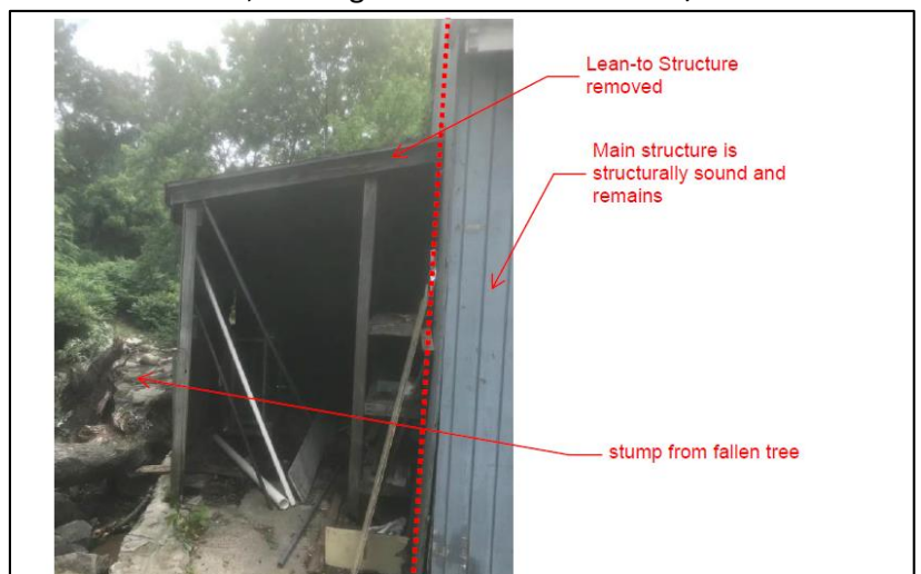
Figure 1 - View looking east at lean toward constructed on stream wall
