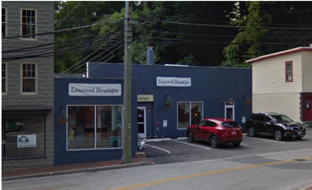
Figure 2 - Front facade showing locations of proposed signs
