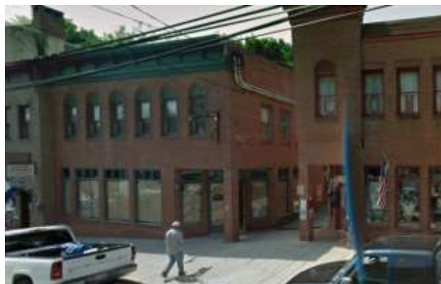
Figure 11 - Alley between buildings
