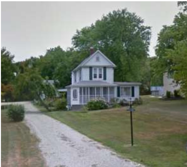
Figure 20 - House to be demolished
