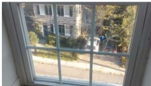
Figure 18 - Dormer window to be replaced
