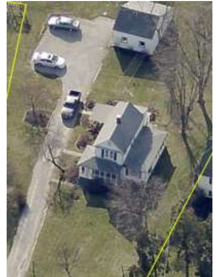
Figure 19 - House to be demolished
