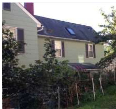
Figure 17 - View of roof
