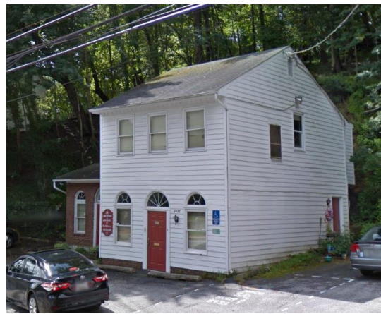
Figure 2 - Front and west side of building
