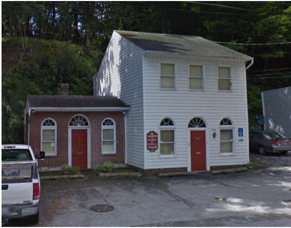
Figure 1 - Front of building
