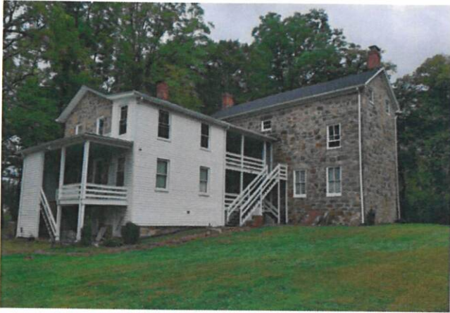
Figure 22 - Rear of house, facing Knoll Glen Drive.
