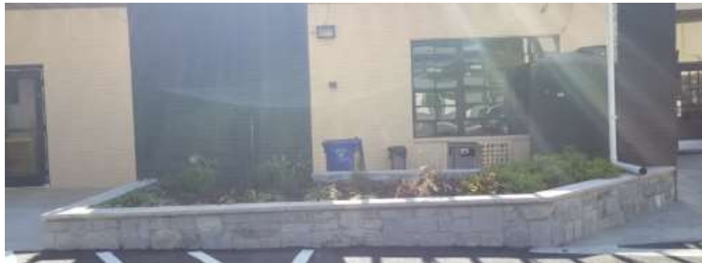
Figure 11 - Approved replacement wall from August 2016
