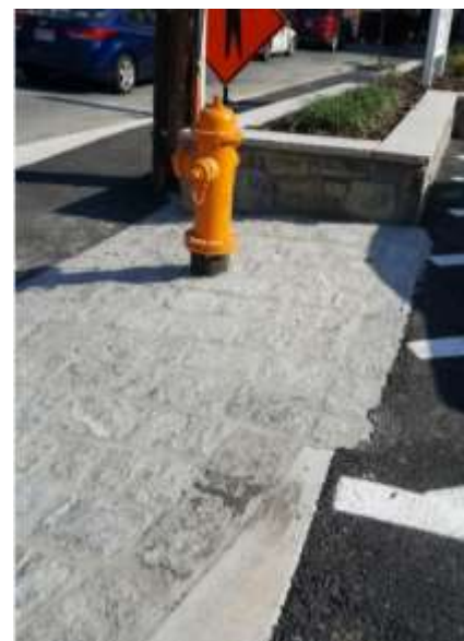
Figure 8 - Granite cobblestone pavers installed
