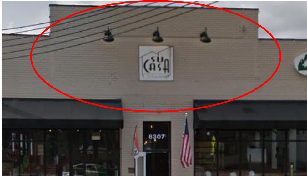
Figure 5 - Defined brick area on facade
