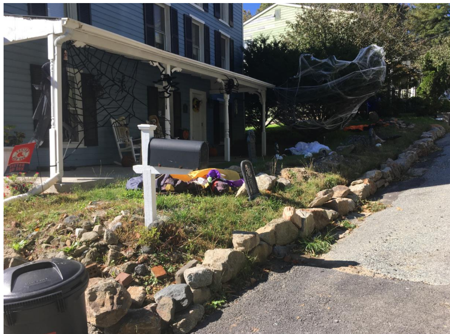
Figure 21 - View of partially built wall along property and street
