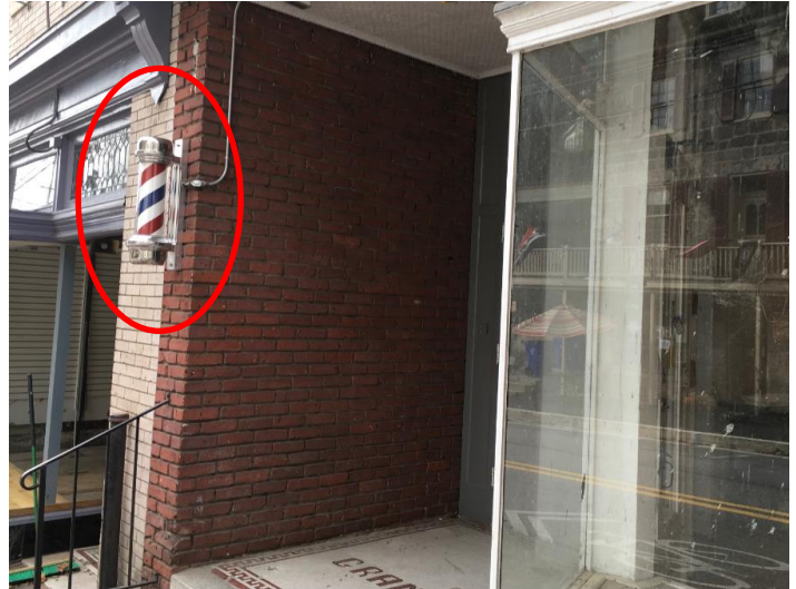
Figure 24 - Location of barber shop pole
