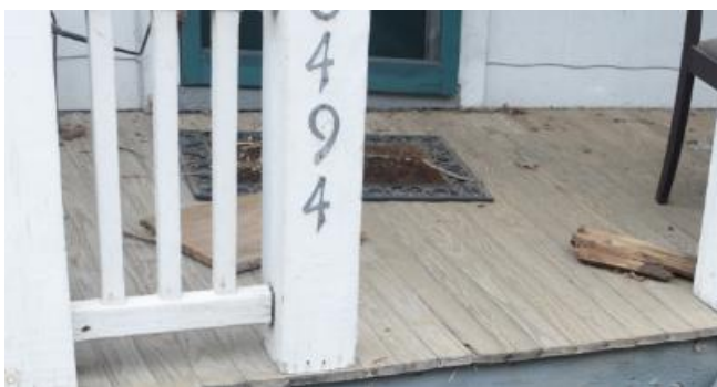
Figure 10 - Existing porch flooring/decking
