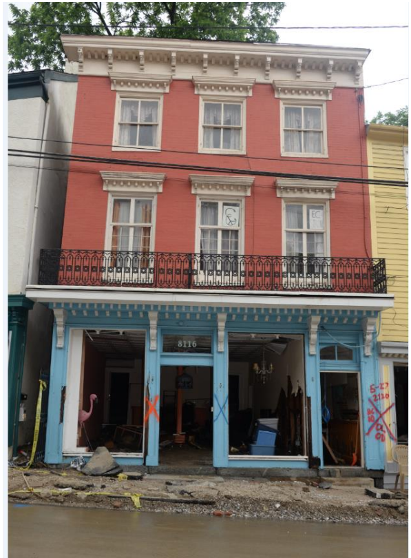
Figure 2 - Damage from 2018 flood
