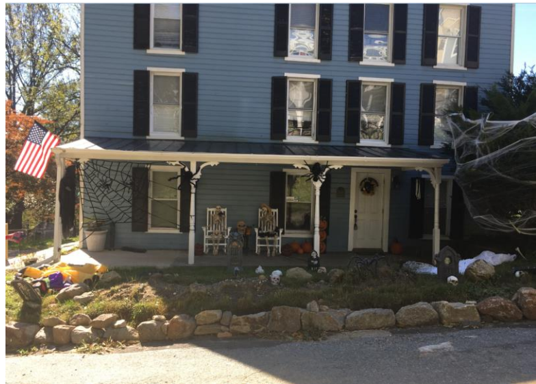
Figure 20 - Front view of house and partially built wall
