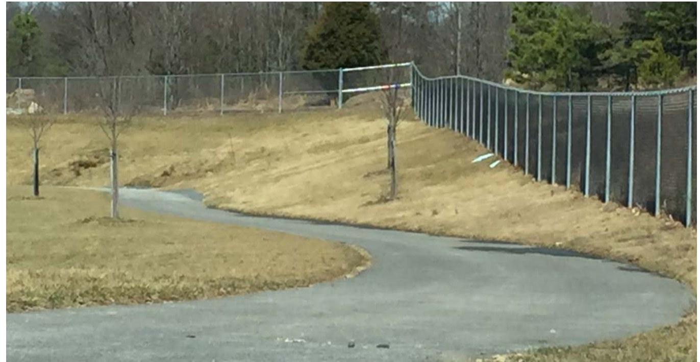
Shared-Use Path at Middle School (February 2016)
