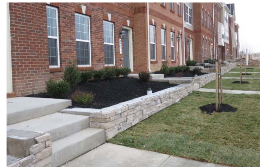
Bio-Retention at Oxford Square
