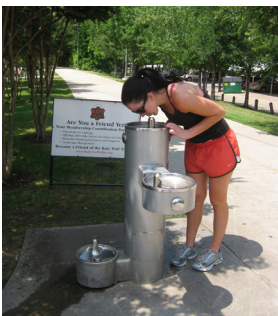
Drinking Fountain Source: TDG Library
