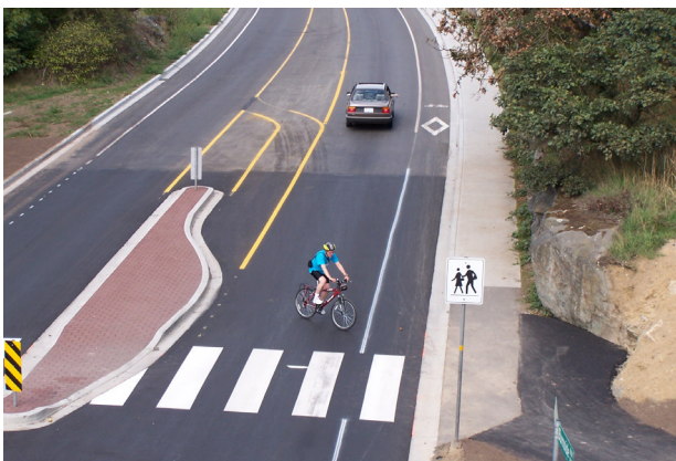
Intersection Crossing Source: TDG Library
