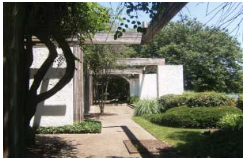
East Facade, with Lake Level Terrace
