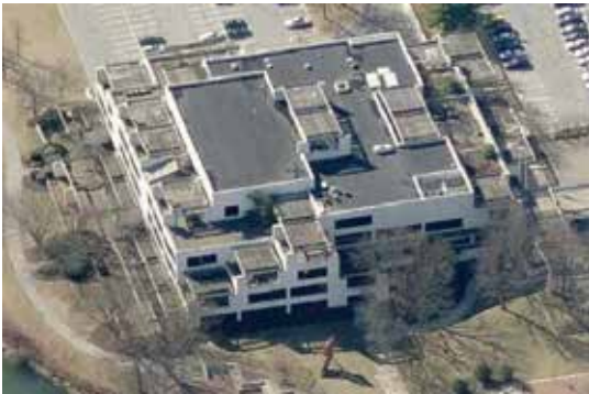
Overhead view from North-East
