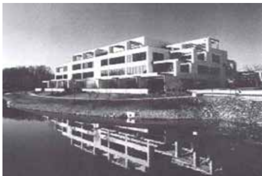
View from North-East
