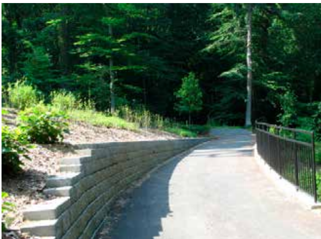
Segmented Concrete Retaining Wall Source: TDG Library
