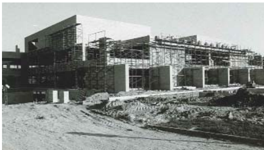
Concrete masonry unit solid walls
