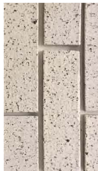
BRICK SYSTEM - SOUTH ENTRANCE ROAD
