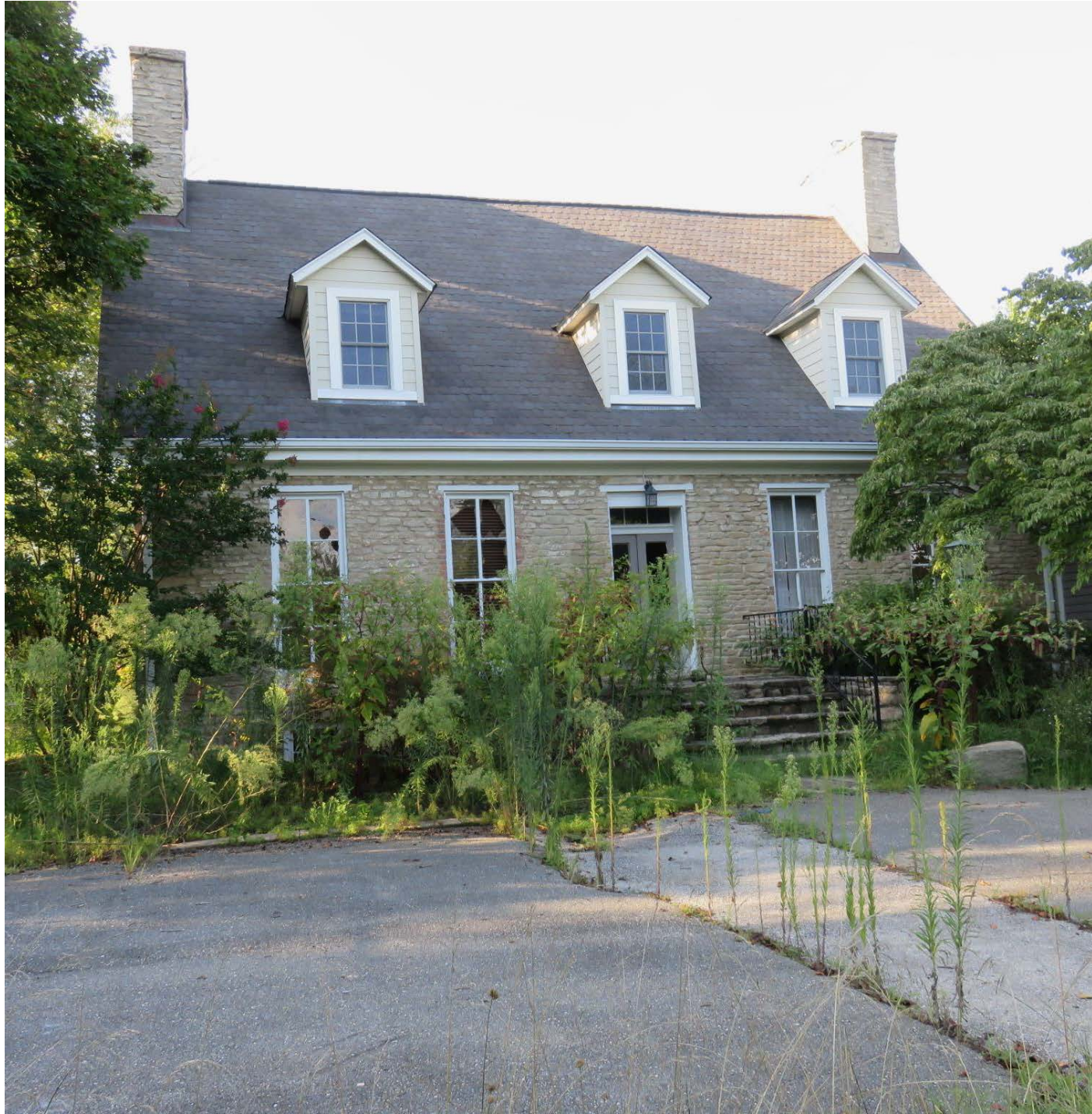
ATHOL MANOR HOUSE (FRONT VIEW)
