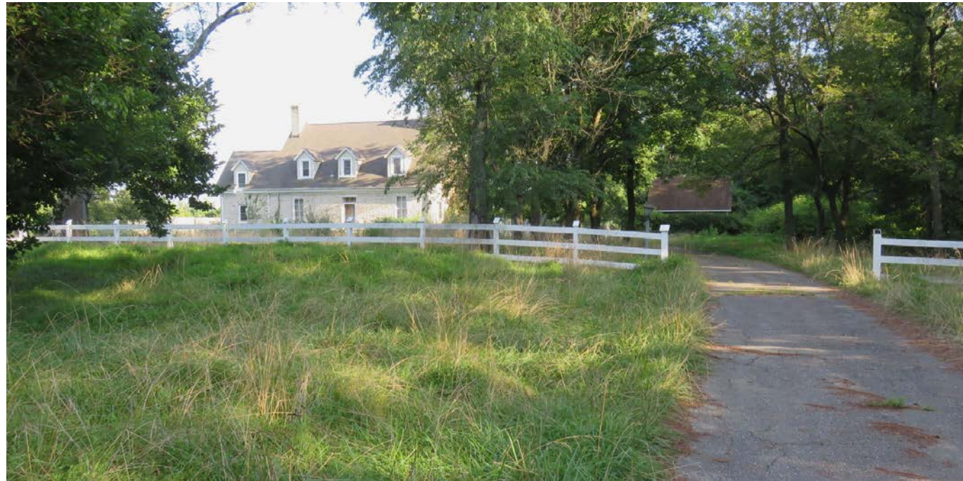
ATHOL MANOR APPROACH FROM THE NORTH
