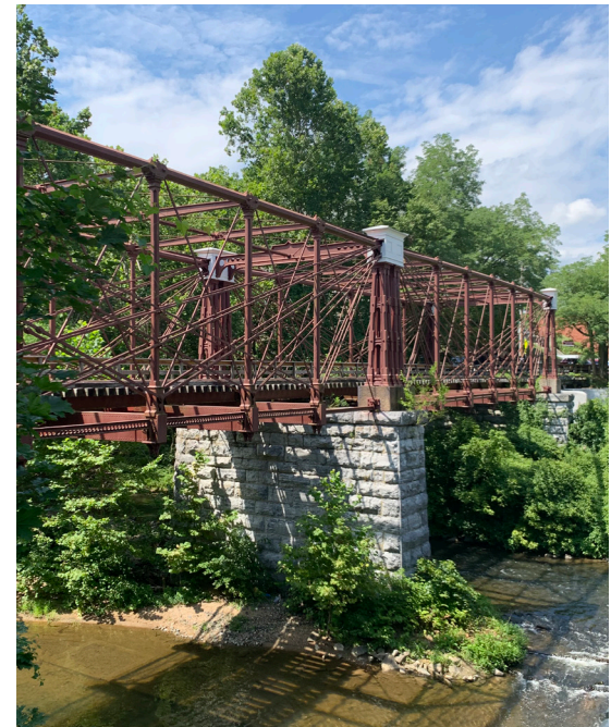
Figure 141: Savage Mill Trail Connects Neighborhoods to Downtown Savage
