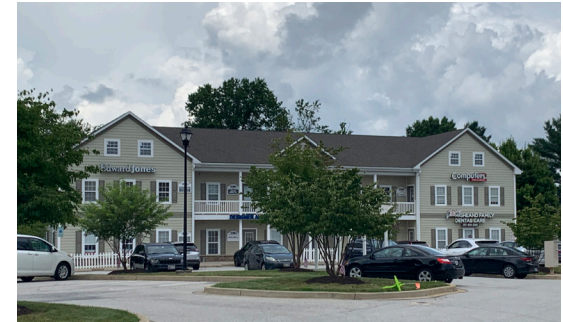
Figure 63: Small-Scale Office Center in Highland
