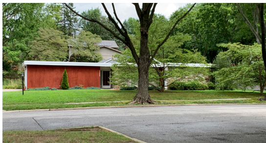
Figure 82: Early Contemporary Architecture within Suburban Neighborhood
