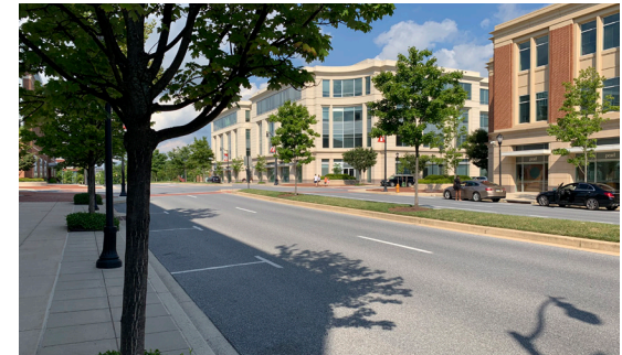
Figure 154: Streetscape at Maple Lawn
