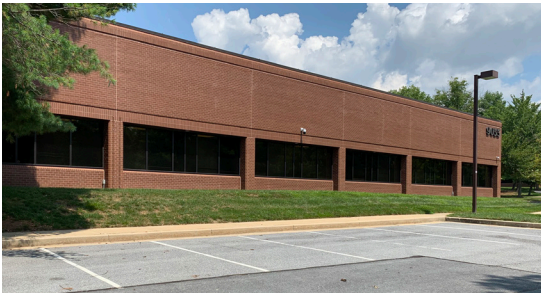
Figure 187: Single Story Modernist Office Building in Gateway
