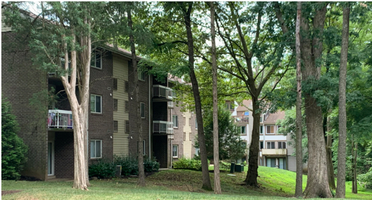
Figure 94: Typical Older Apartment Neighborhood Organized Around Open Space
