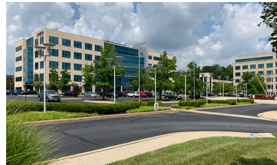
Figure 123: Gateway Corporate Park Office Cluster
