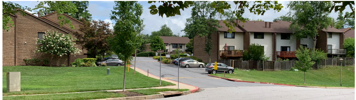
Figure 97: Typical Older Townhouse Neighborhood
