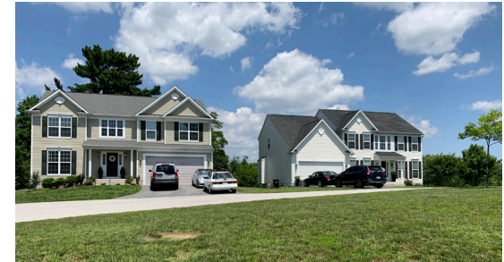
Figure 84: New Construction within Suburban Neighborhood
