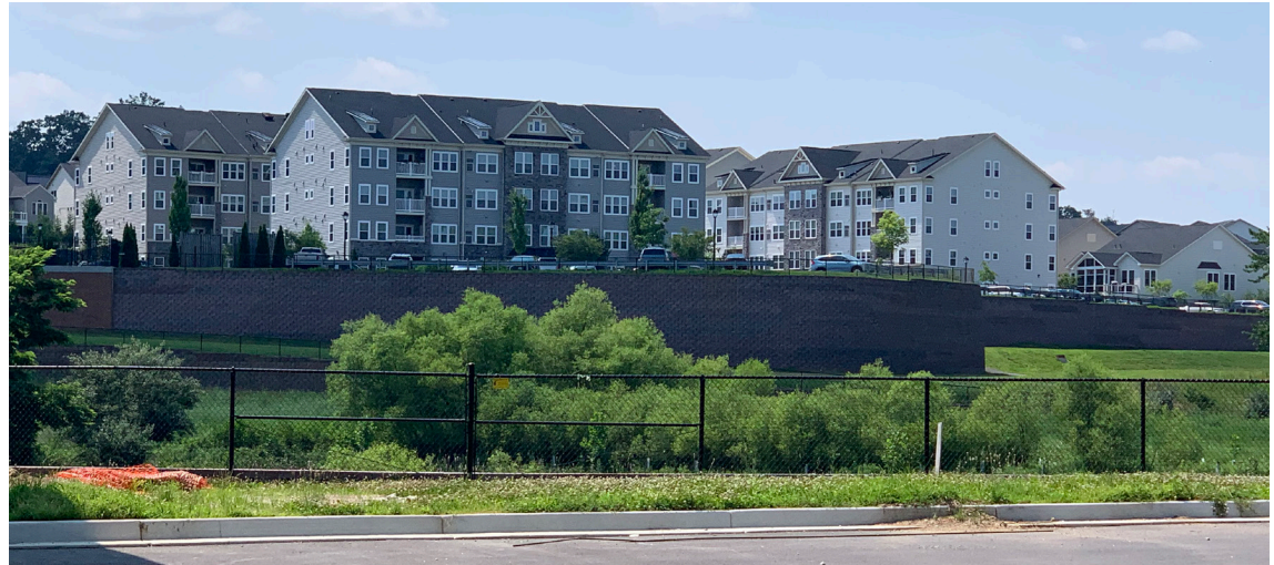
Figure 183: Example of the Land Adapted to Fit the Buildings vs. Buildings Designed to Fit the Land
