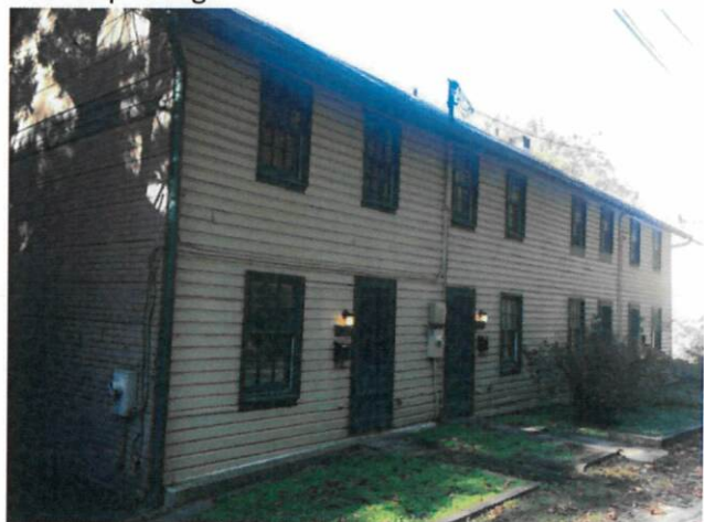
Figure 6 - Front facade of one set of buildings showing German lap siding and brickmold shingles.
