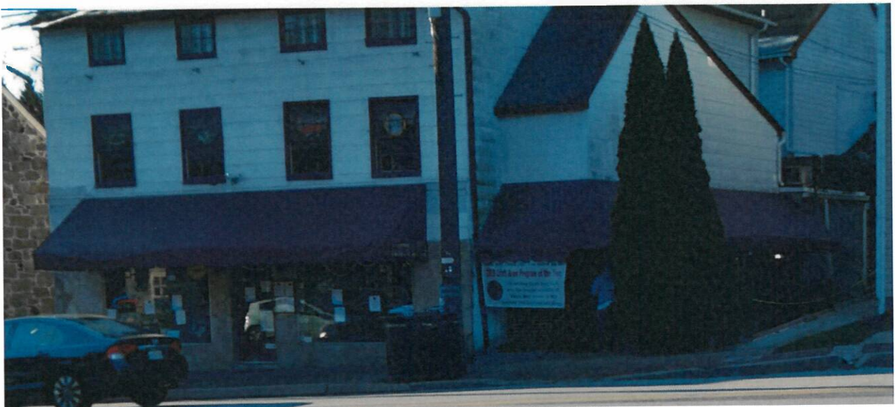
Figure 9 - Existing conditions. Awning on right side to be replaced. Front awning to remain.
