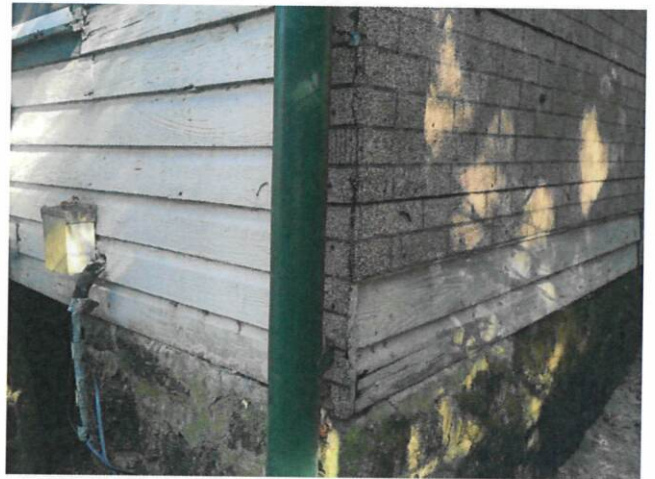
Figure 7 - Existing German lap siding, brick mold shingle and German lap siding under brick mold shingle.
