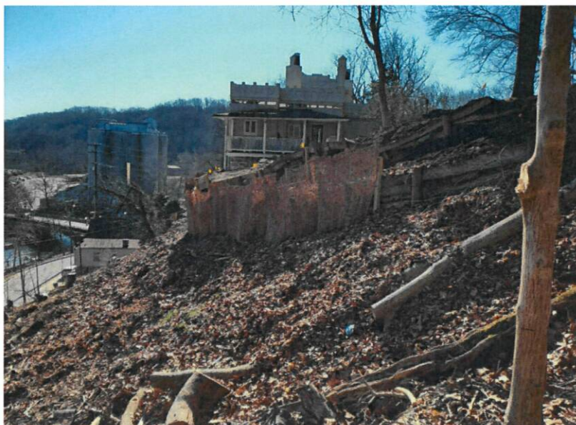
Figure 17 - Conditions in January 2020
