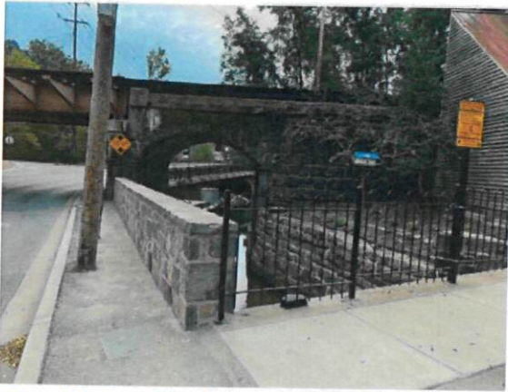
Figure 11 - Area of replacement parallel to Main Street
