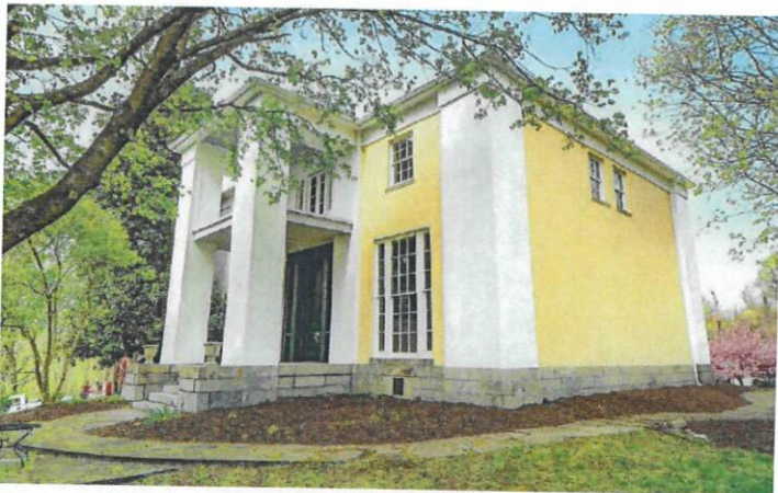
Figure 4 - Southeast elevation facing Church Road
