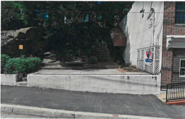
Figure 9 - Before fence was installed.
