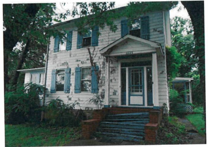
Figure 4 - 6925 Linden Avenue, to be demolished.
