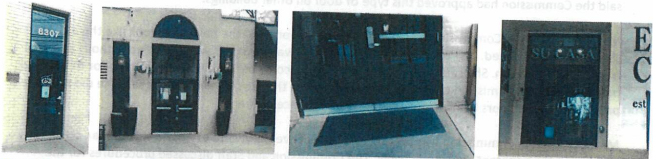
Figure 37 - Current doors on 8307 Main Street
