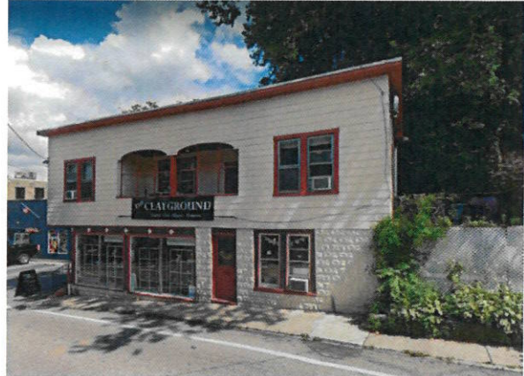
Figure 13 - Front facade along Old Columbia Pike.
