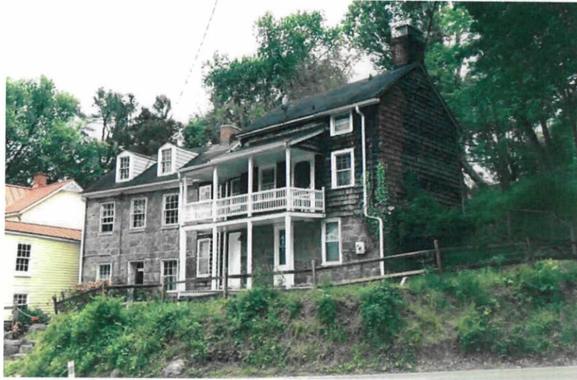
Figure 16 - Existing front facade view from Old Columbia Pike. Three-bay wide stone house to the left is a separate residence.
