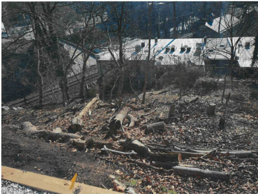
Figure 19 - Site conditions in January 2020. Looking south east toward Main Street (buildings in background front Main Street, the B&O is visible, front Maryland Avenue) and train tracks.
