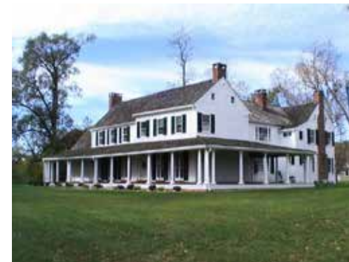
RICHLAND, CLARKSVILLE – white lap siding, gable roofs, divided-lite windows
