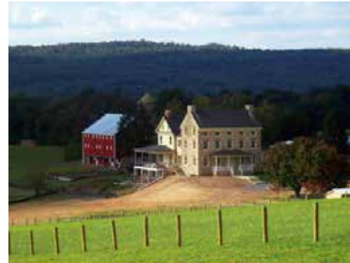
MONTGOMERY COUNTY HOUSE – hipped roof porches, masonry and siding
