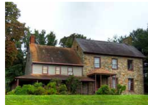
CARROLL COUNTY HOUSE – masonry and siding, window surrounds, gable roof
