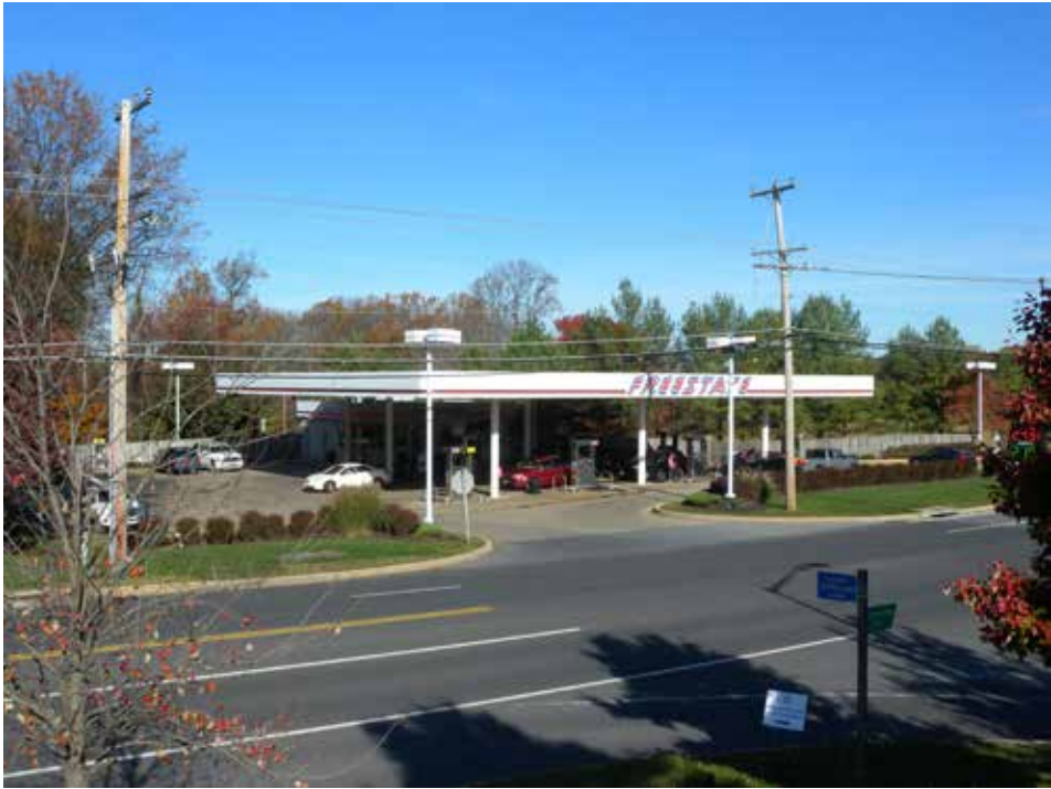
FREESTATE GAS STATION
