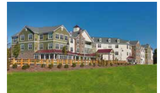
masonry and siding composition, red metal roofs, roof dormers, cupola
