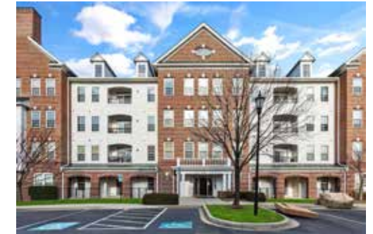
THE VILLAS AT RIVER HILL, CLARKSVILLE – brick masonry and siding composition, roof dormers, metal roofs
