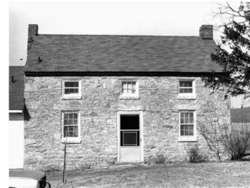
LIMESTONE VALLEY FARM STONE TENANT HOUSE, CLARKSVILLE – stone masonry, gable roof, divided-lite windows
