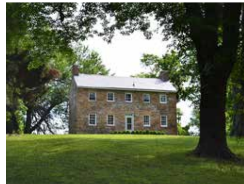
IVY HILL, MARIOTTSVILLE – masonry, gable roof, divided-lite windows
