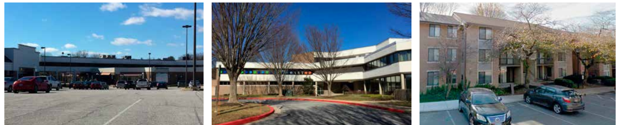
Existing Site Photos (Above)
