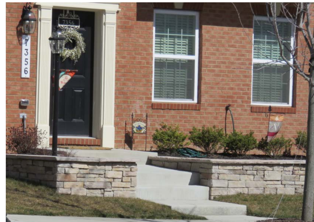
Residential Site Walls (along St. Margaret's Boulevard)
