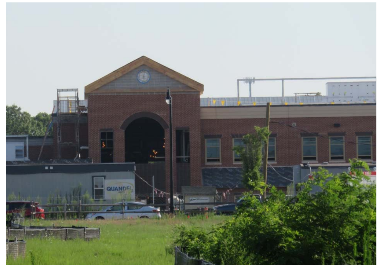
4. Elementary School Under Construction (Summer 2017)
