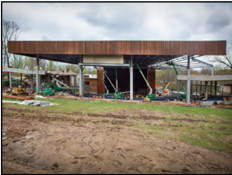
The MPP renovations include a new, higher roof (shown above) and new office and backstage areas.
