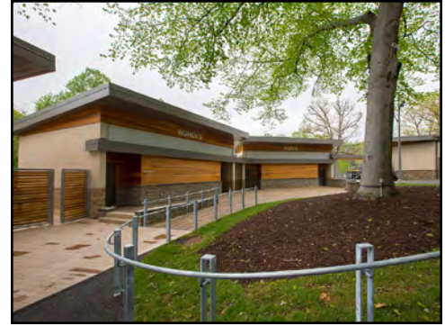
New Restrooms at Merriweather Post Pavilion
