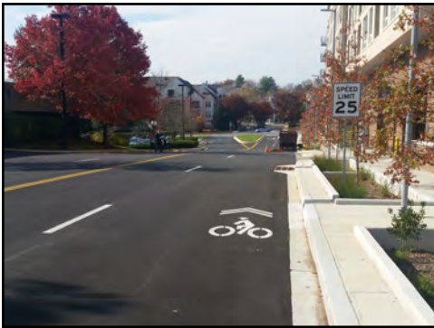
Sharrows on Grammercy Place are an example of a Complete Streets provision.
