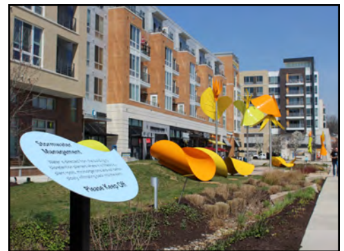
Bioretention planter at The Metropolitan
