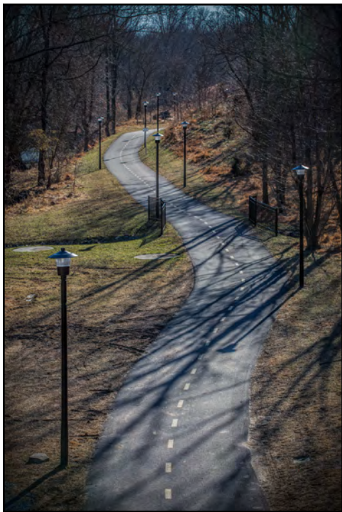
The Downtown Columbia Trail uses permeable asphalt to allow stormwater to infiltrate.
