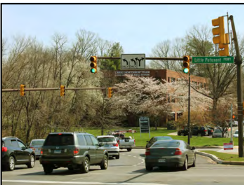
A third left turn lane was added to Governor Warfield Parkway at Little Patuxent Parkway.
