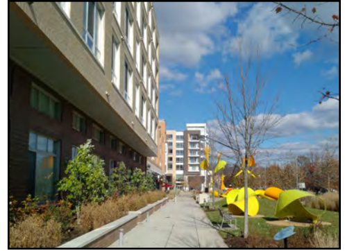
New Sidewalk at The Metropolitan
