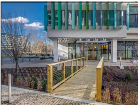
Crescent Area 1 features a large rain garden adjacent to Two Merriweather.
