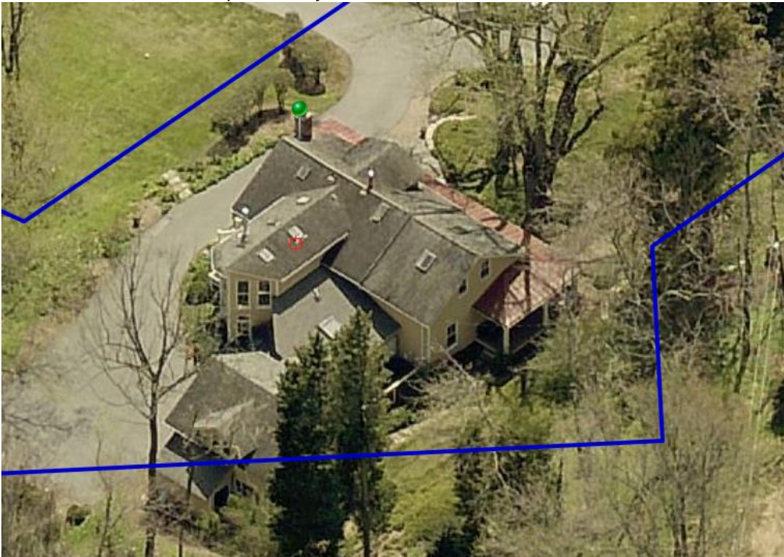
8390 Park Drive, Ellicott City: Roof Project
