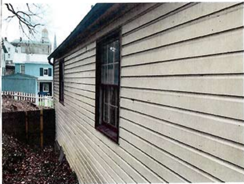
Rear of building to be painted same colors
