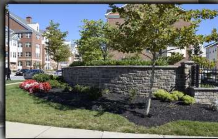
Site Landscape Walls
