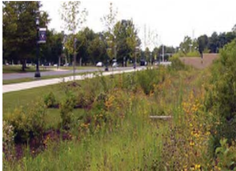
Bioswale along street
