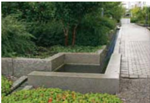
Rainwater is drained into the canal from the surrounding buildings via gutter planter as water feature.
