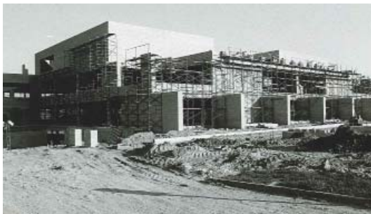
Concrete masonry unit solid walls
