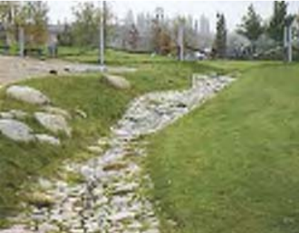
Example of surface Bioswale
