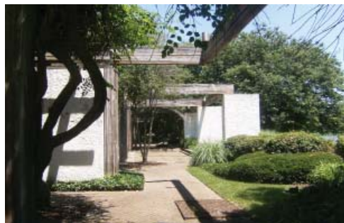
East Facade, with Lake Level Terrace
