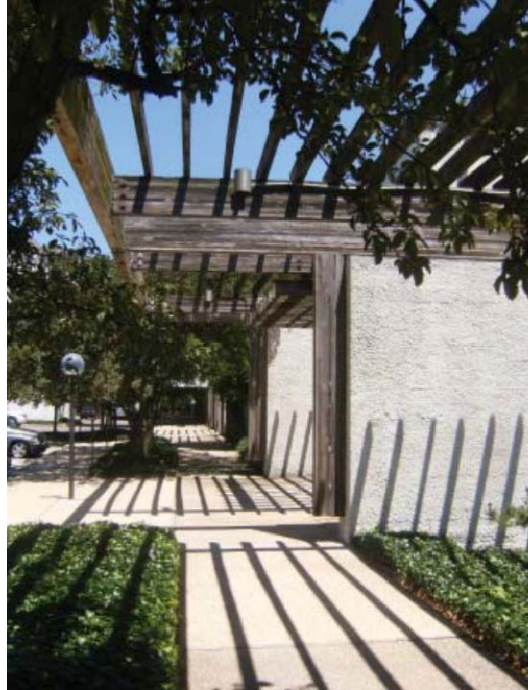
Wood Trellis at West Facade
