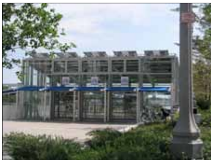
Bicycle Parking Facility
