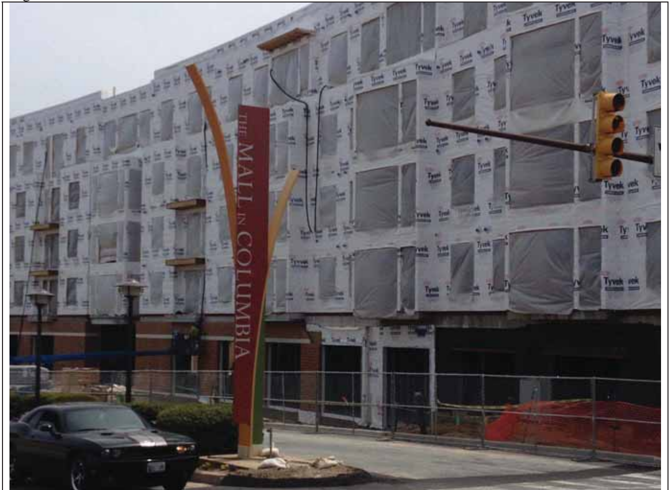
Construction of “The Metropolitan” seen from this vehicular entrance to the mall helps to illustrate the changes coming to Downtown Columbia
