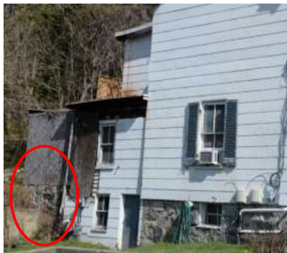
Figure 39 - Existing stone foundation
