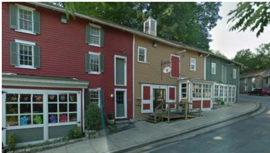
Figure 26 - Front of building before renovations
