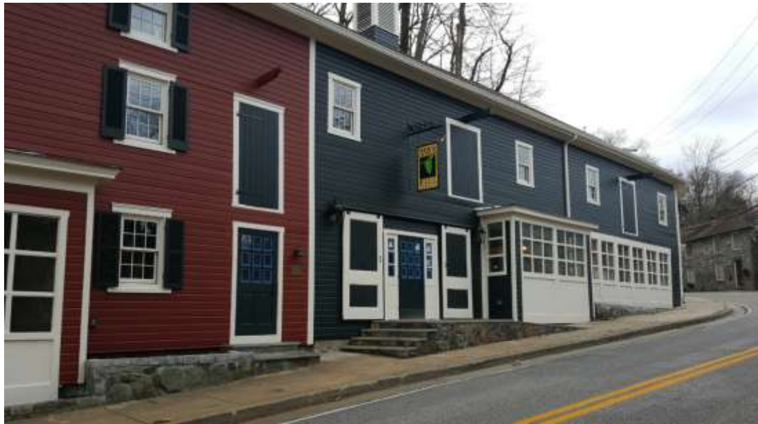
Figure 234 - Front of building after renovations
