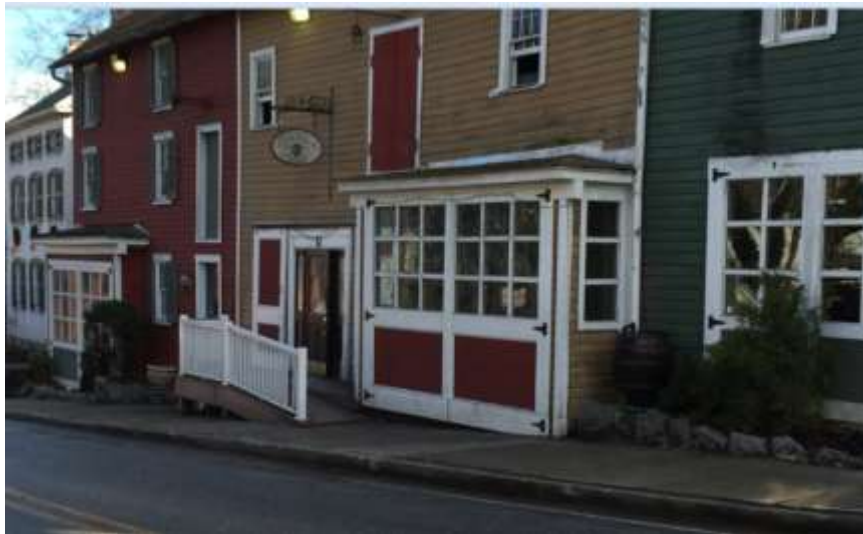
Figure 25 - Front of building before renovations
