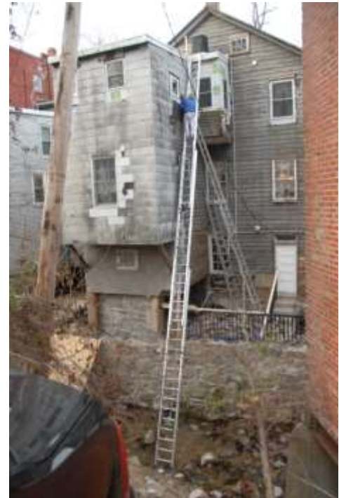
Figure 32 - Asbestos siding being removed
