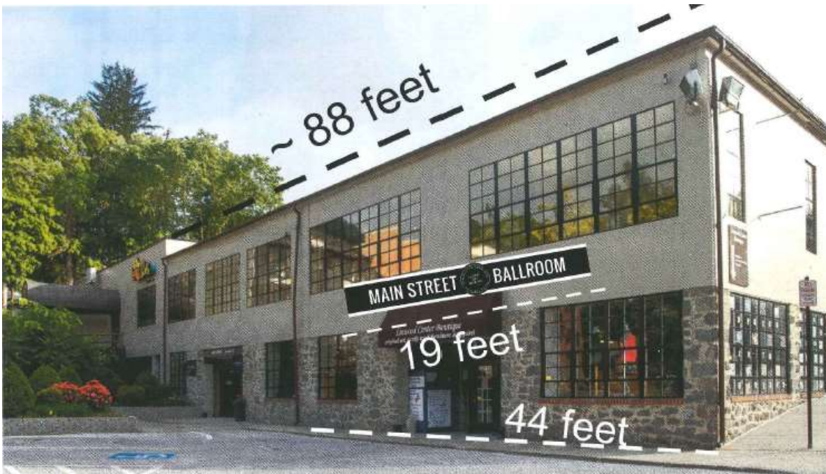
Figure 29 - Rear of building
