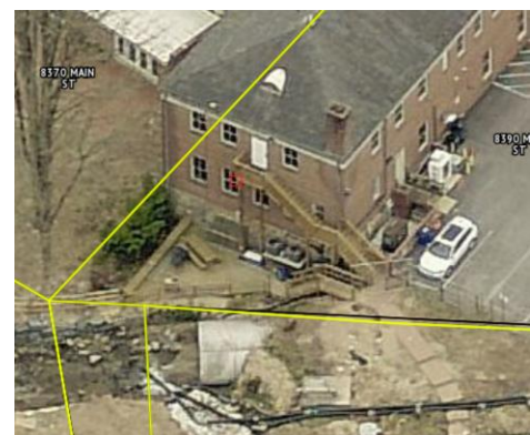
Figure 38 - Aerial view of the rear of the building.
