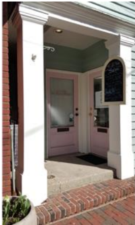
Figure 26 - Doors in April 2016
