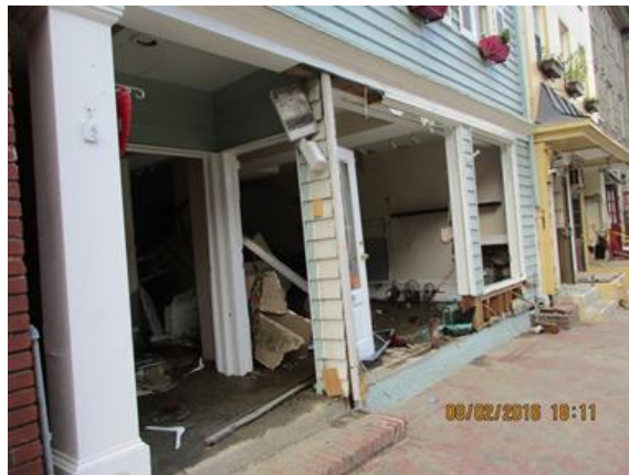
Figure 27 - Damage from 2016 flood
