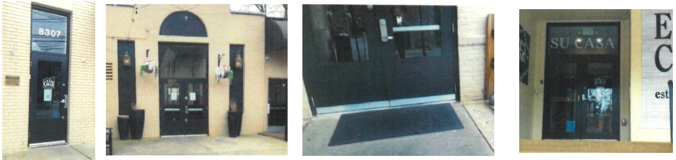
Figure 37 - Current doors on 8307 Main Street
