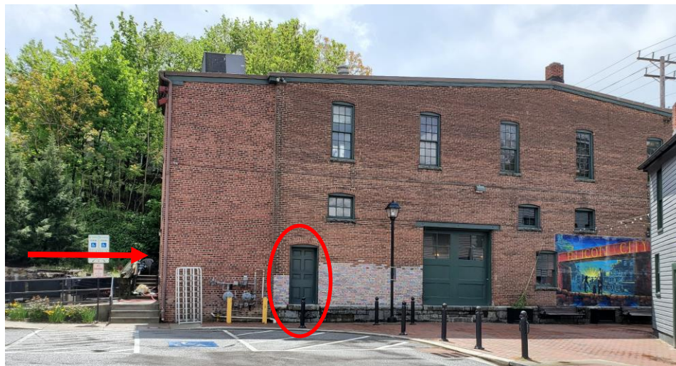
Figure 15 - Red arrow points to rear metal door and red circle shows side door. Please note – the colored brick around the red circle is only chalk.
