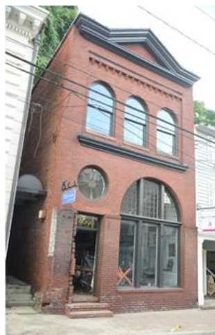
Figure 30 - Damage from 2016 flood
