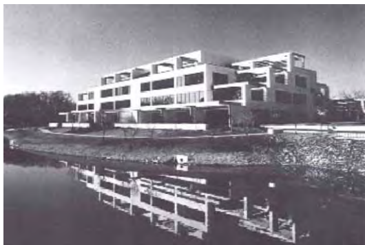
View from North-East
