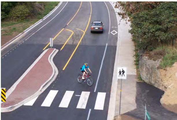
Intersection Crossing Source: TDG Library
