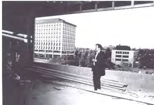
Frank Gehry inspects construction site
