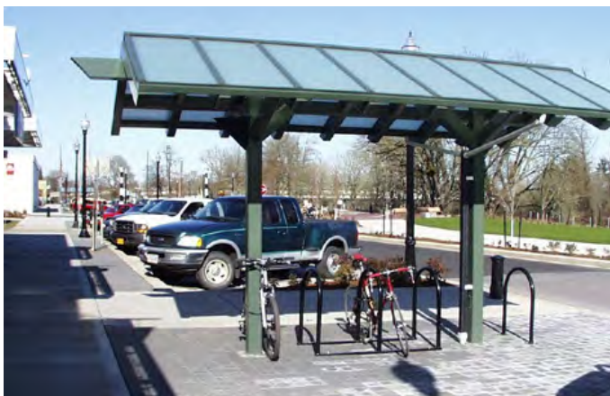
Covered Shelter Bicycle Parking Source: TDG Library
