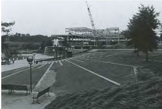
Steel framed building structure, under construction
