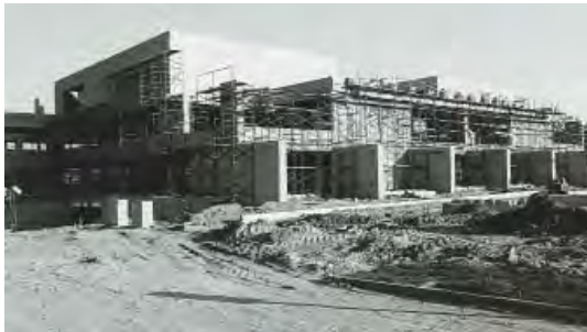
Concrete masonry unit solid walls
