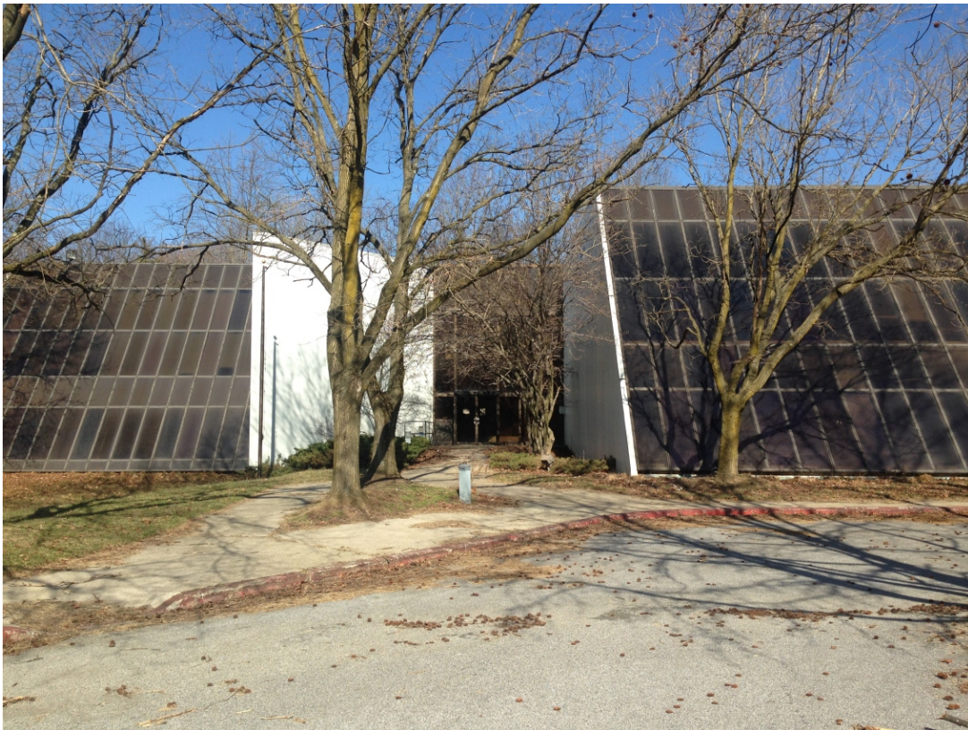
Photo 2: View of the eastern portion of the on-site building looking from east to west.
