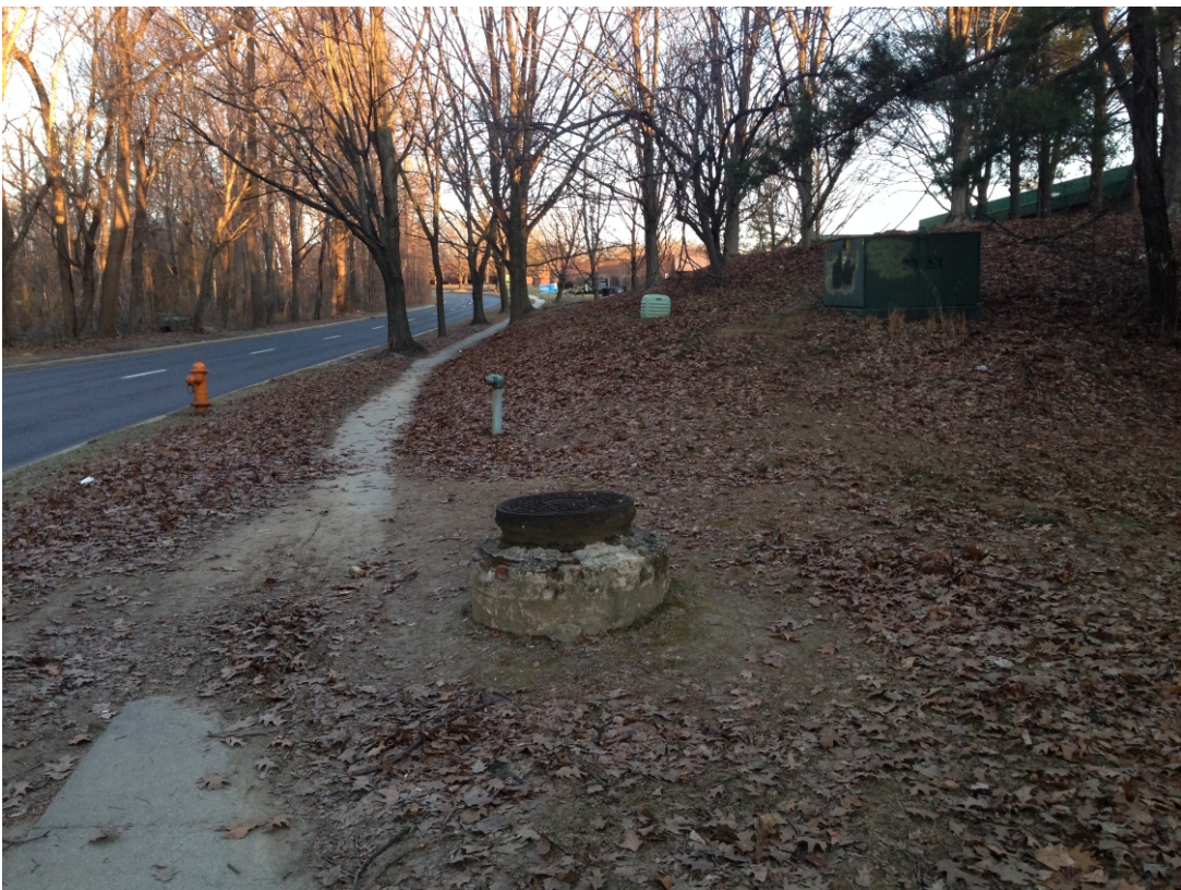
Photo 6: View of the public utilities located along the southern portion of the site.
