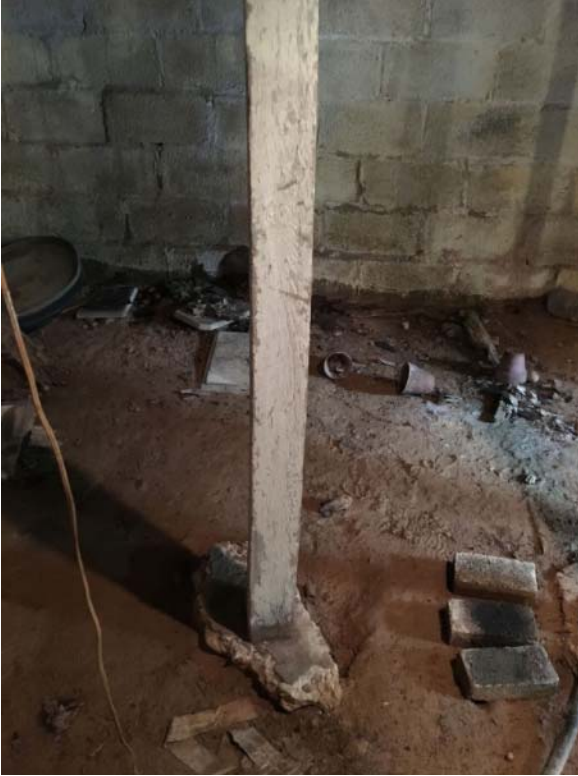
Existing wood column, currently set on concrete remnant
