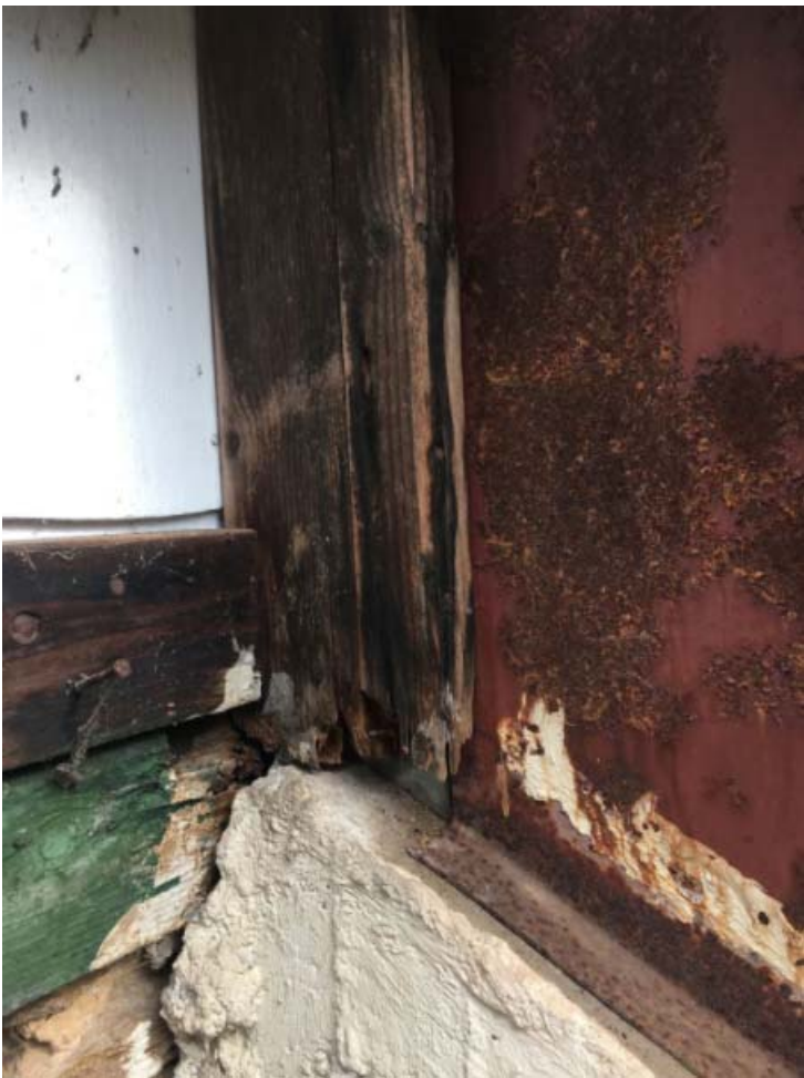
View of wood frame top right of Bilco door
