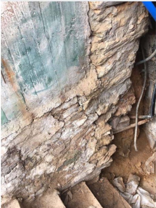
Foundation wall left wall near exit
