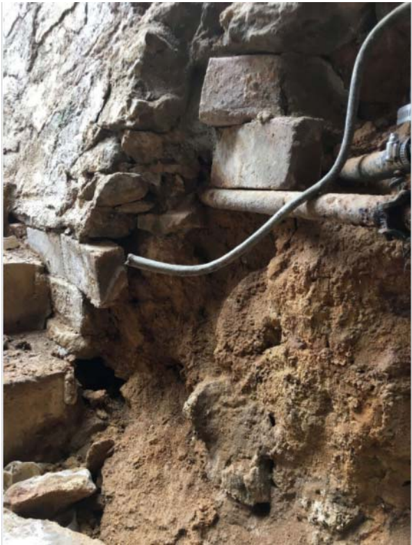
Foundation wall near exit
