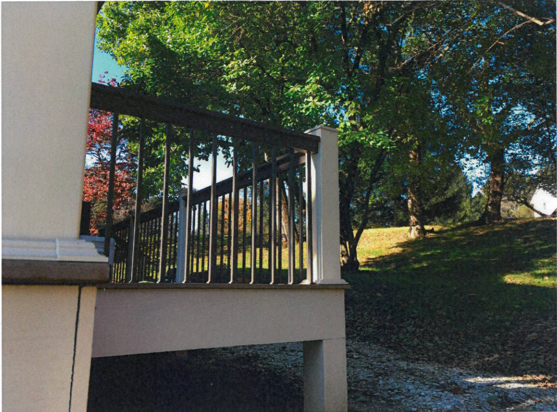
View of 3820 Old Columbia Pike from Road. Deck not in view
