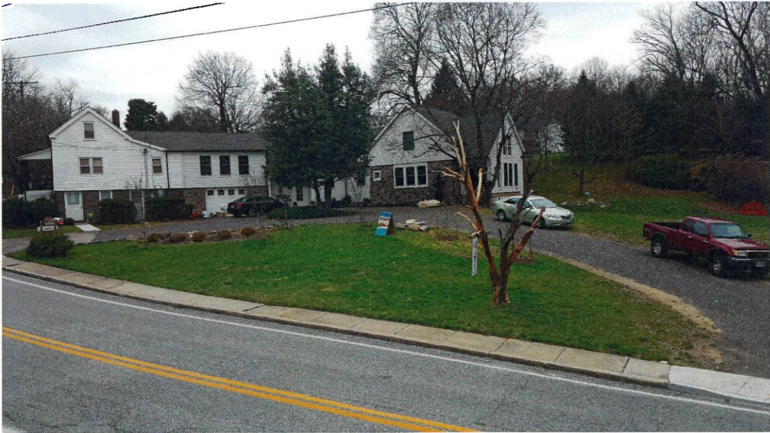
View of current PVC deck post sleeves to be replaced with aluminum with BEHR paint Mushroom Bisque
