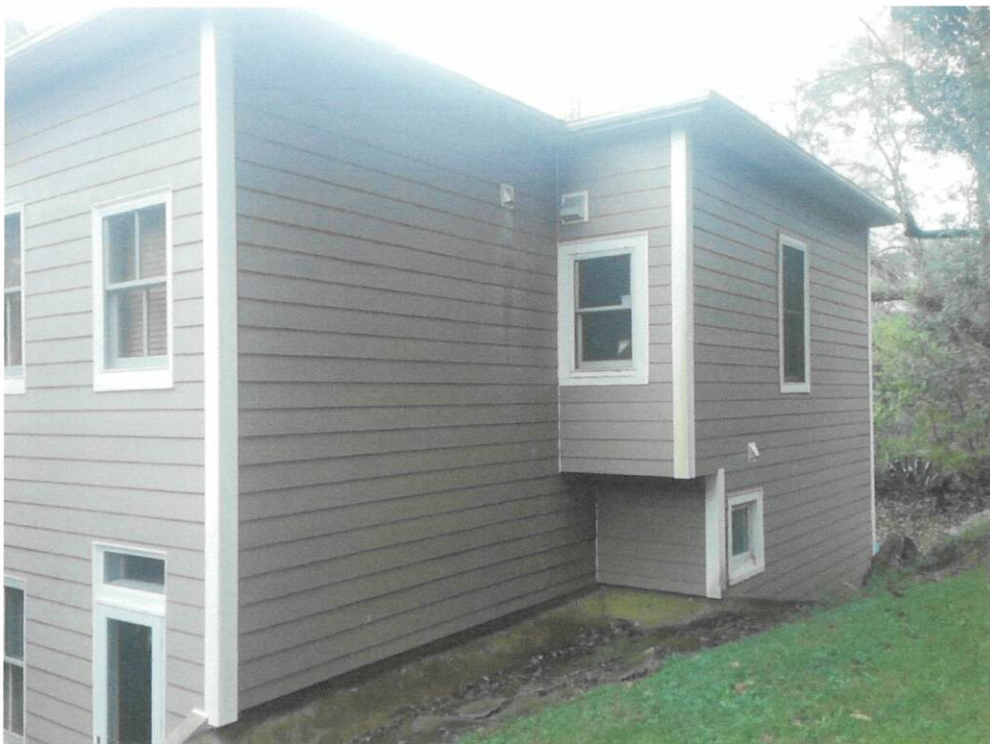
Rear of House
