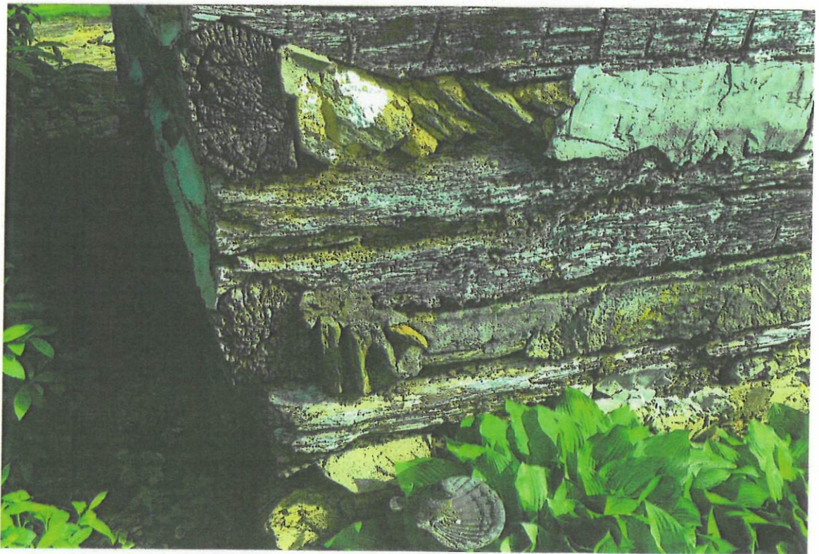
FRONT (SOUTH SIDE)
