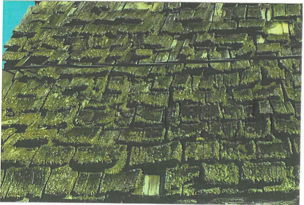
CEDAR SHAKE ROOF
