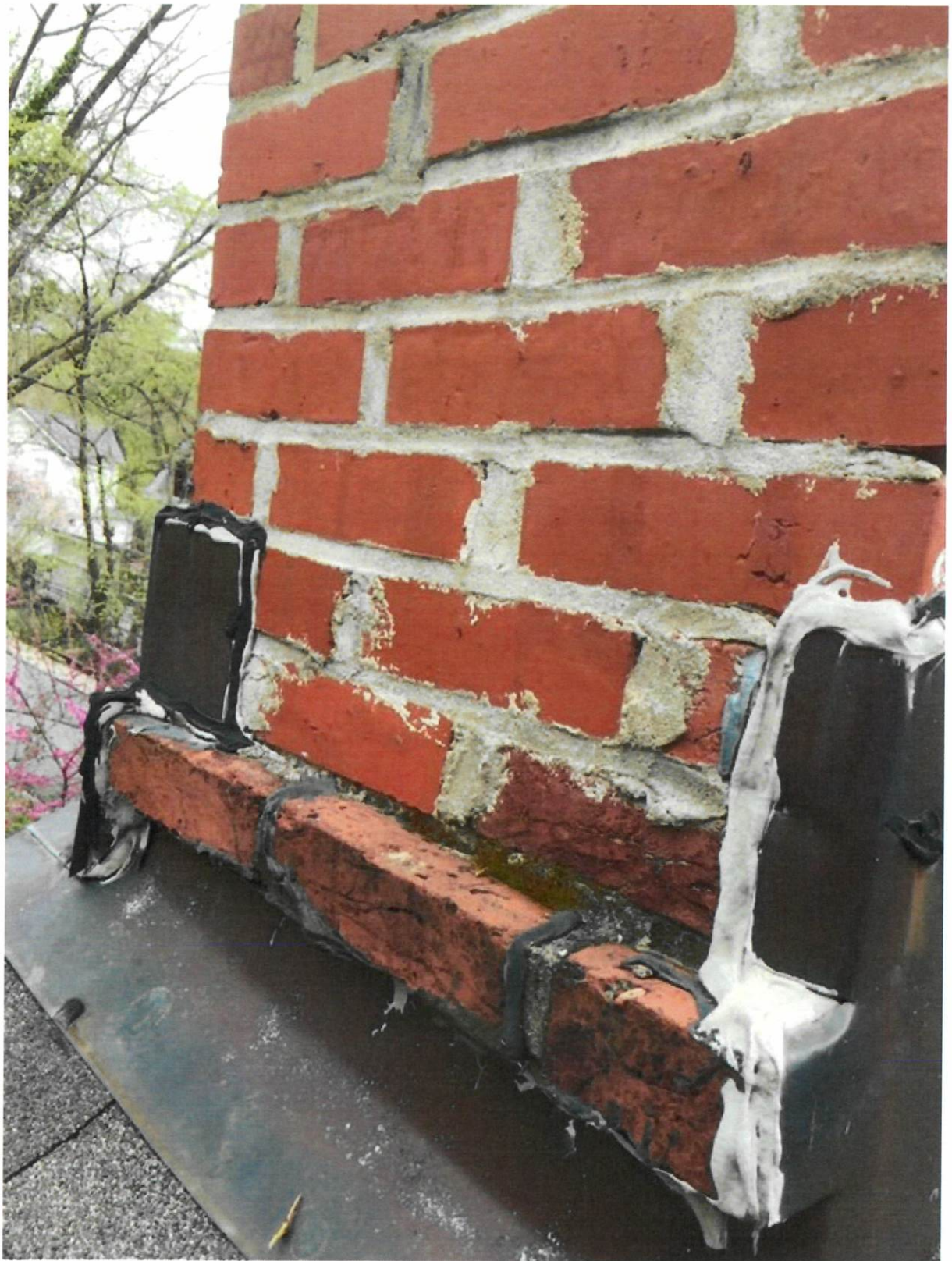
Chimney Backside (facing rear of house)
