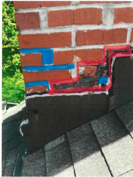
Chimney Sideview (facing summer kitchen)
