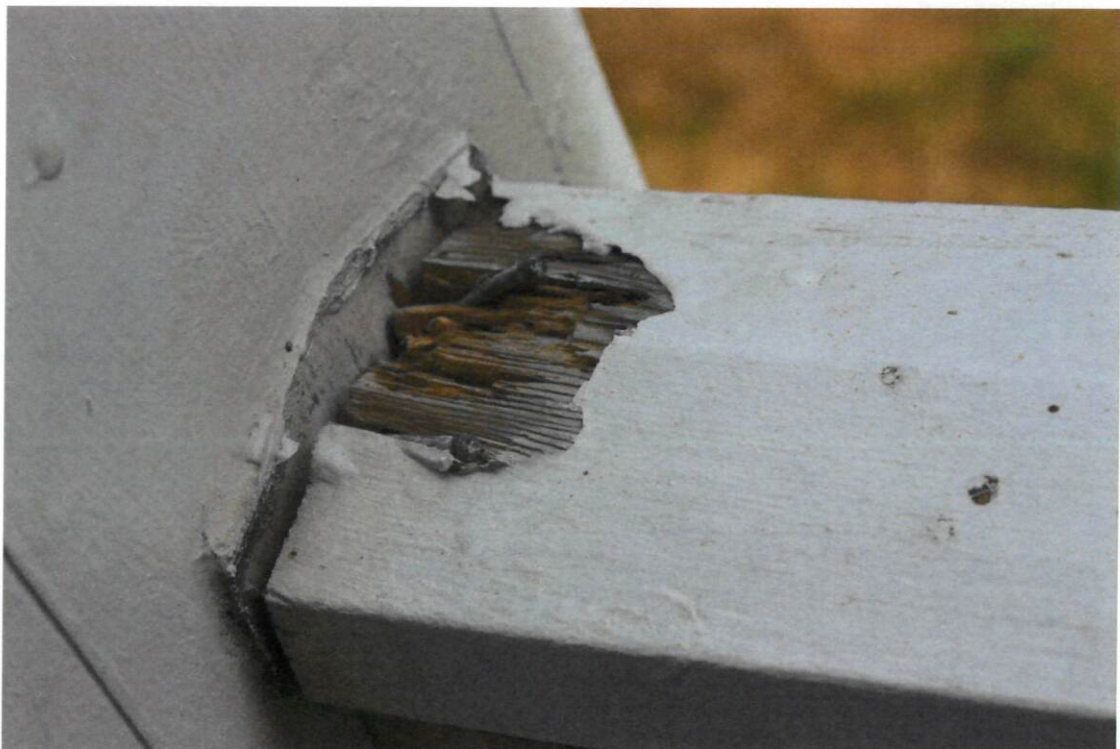
Photo 4 – Rotting railing
