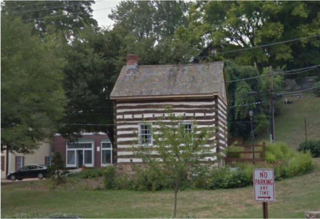
NORTH (REAR) SIDE OF CABIN
