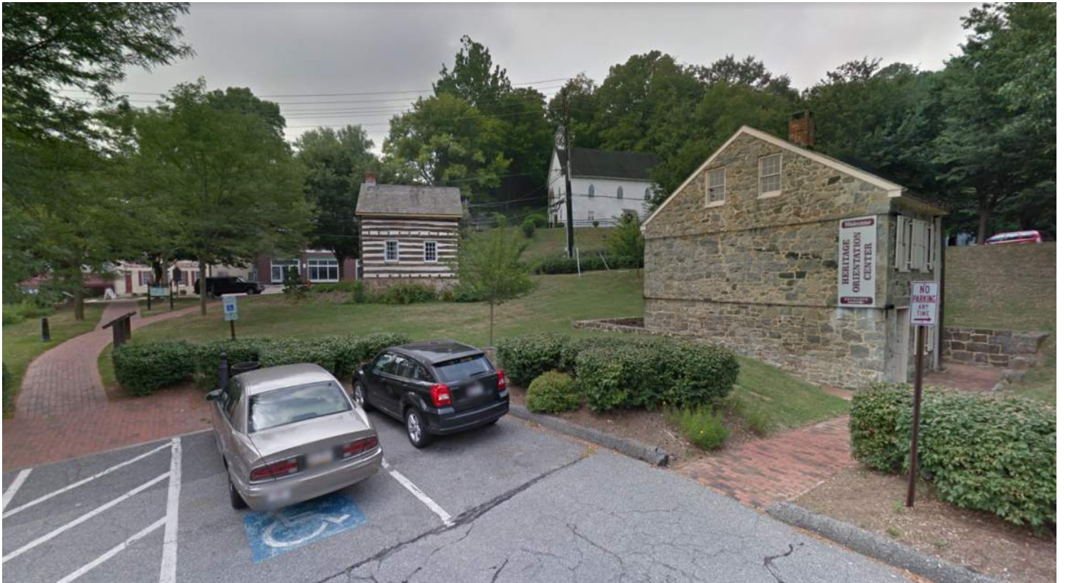
NORTH SIDE OF CABIN FROM PARKING LOT
