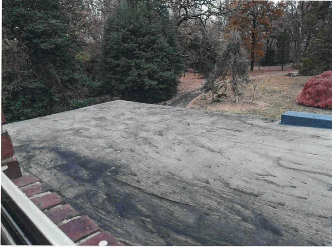
Front porch roof from 2nd floor window.
