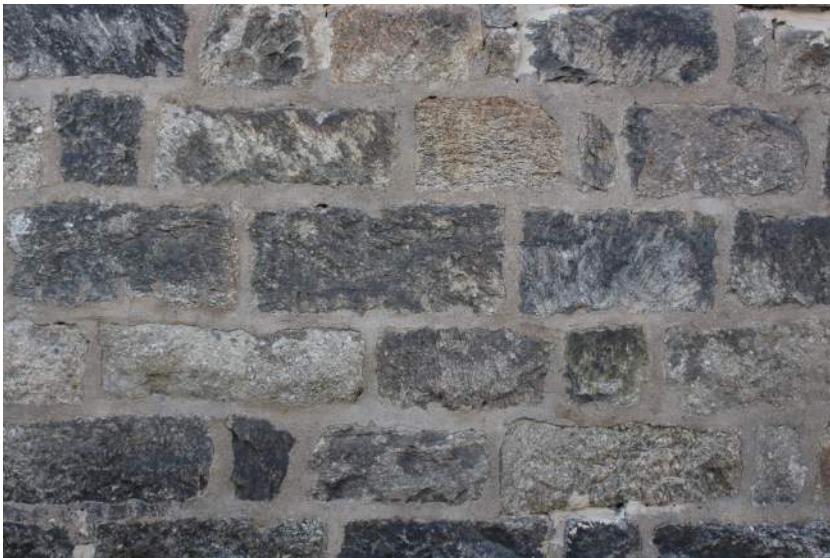
Image 5.3 - Mortar "Type A" - in good condition
